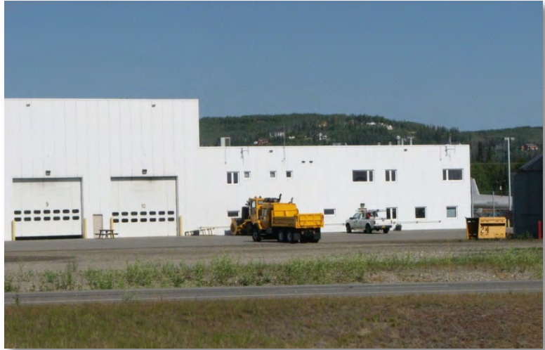
Figure 2-36 – ADOT&PF Maintenance Facility
