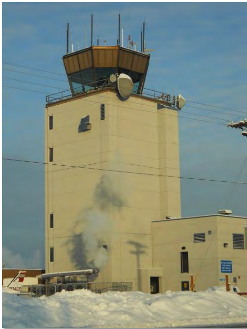
Figure 2-40 – FAI Air Traffic Control Tower
