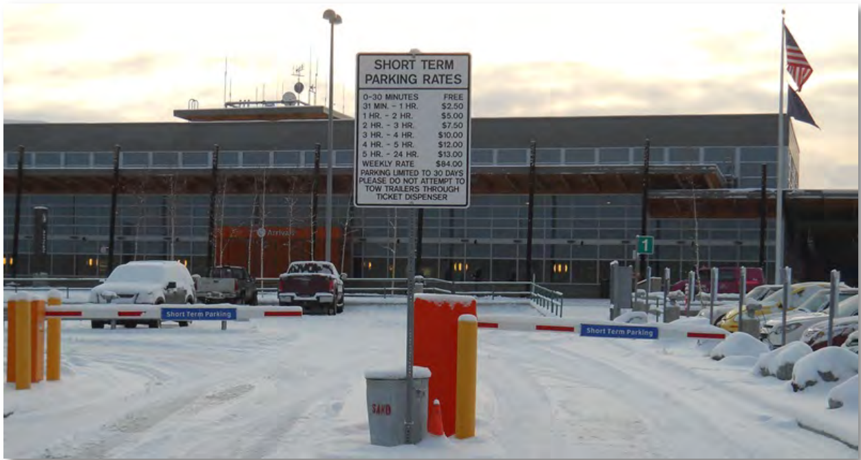
Figure 2-15 – Short-term public parking entrance adjacent to the FAI terminal building
