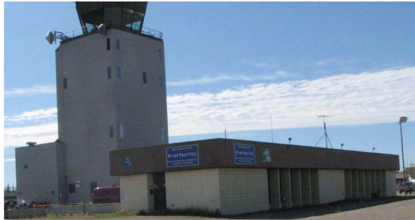
Figure 2-7 – East Ramp pilot facilities
