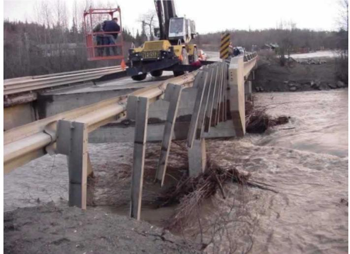
**Project Description:** Description: Install monitoring and telemetry, perform activities required to meet the National Bridge Inspection Standards (NBIS) for scour, implement the DOT&PF Plan of Action (POA) for scour-critical bridges, coordinate with local agencies on NBIS compliance, and design and construct physical scour countermeasures at State bridges identified as scour critical National Bridge Inspection Standards
