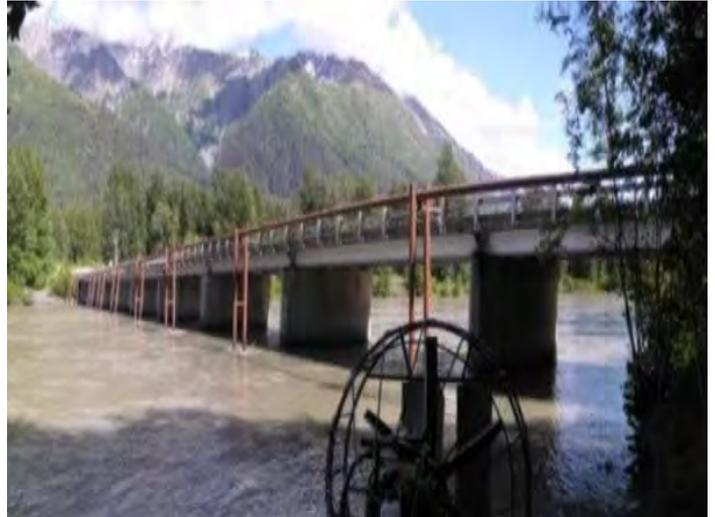
**Project Description:** Replace bridge #742. Possible realignment of road on either side. Widen road to 36'. Straighten curves to meet a 55 mph design speed. Provide a long-term solution to debris flow problems. Enhancements planned along the Chilkat River. This is one of three construction projects that fall under the Haines Highway Reconstruction design project, Need ID 2152. Other construction segments under Need IDs 26330 and 27829.
