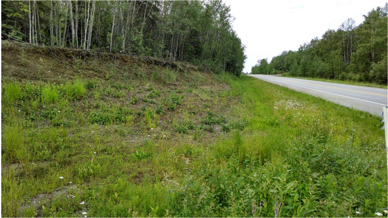
Figure 2-11: Class C soil slope: The soil cut is set back far from the roadway and not affecting structures beyond the ROW. Richardson Hwy MP 319.8.
