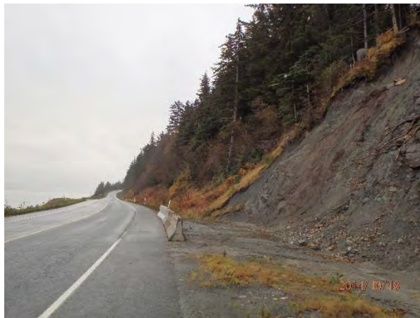
MP 2.21 with concrete barrier
