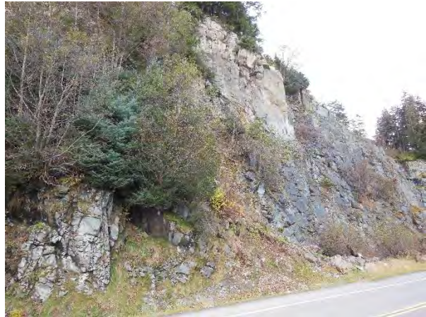
Rock slope at MP 12.81
