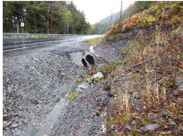
Culverts at MP 5.5
