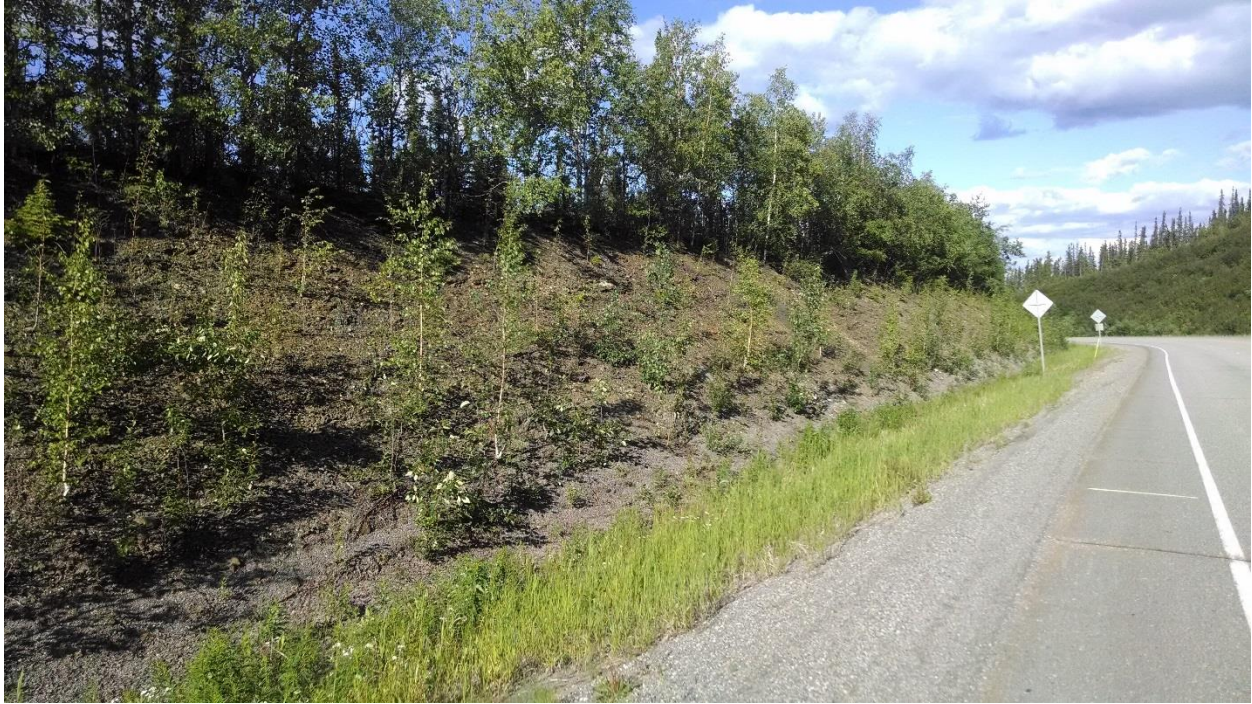
Figure 2-7: Class C rocky slope. Excluded from database due to stable configuration and short height. Either criteria would be sufficient. This could also be reasonably judged a soil slope due to the small rock size. Parks Hwy, approximately MP 340.
