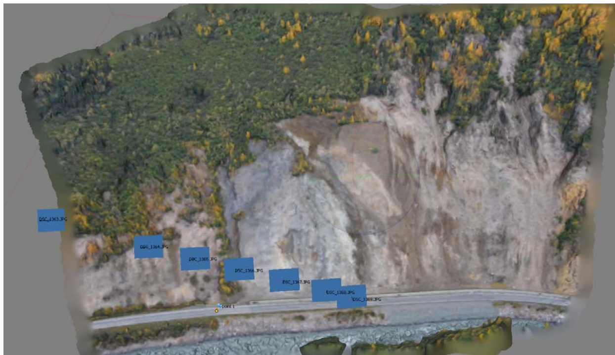
Figure 11-1: Parks Highway PhotoScan surface model. Blue squares indicate helicopter positions. This low density surface consists of 1.6 million points and 323,000 TIN faces.
