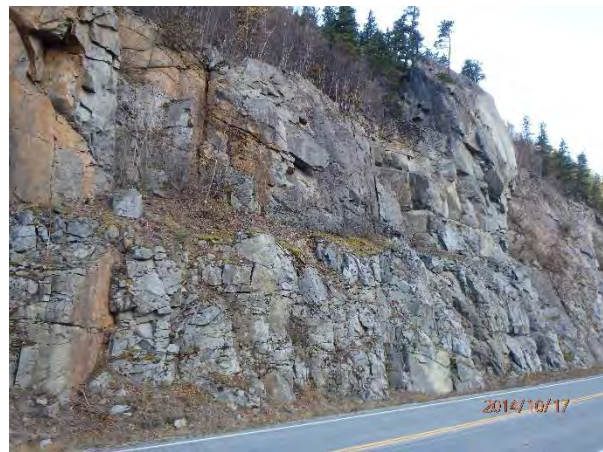
“5-Mile” rock cut
