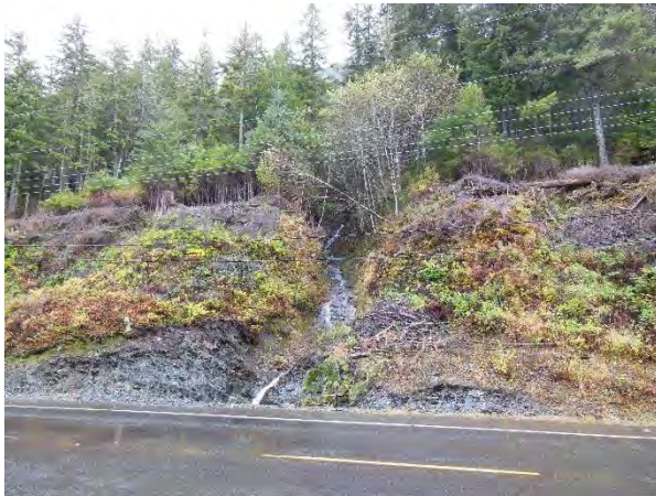
Channel at MP 5.5
