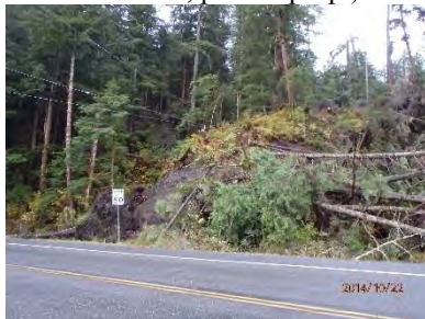
N. Tongass, CDS MP 7.61 (mitigated long landslide with structures and no sign of ongoing movement)
