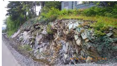
N. Tongass, CDS MP 5.59 (structure above)
