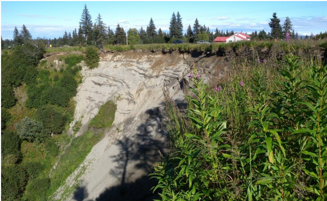
Figure 2-2: Class A soil slope. Slope is receding towards roadway due to piping around spring at base of slope. Sterling Hwy MP 153.3.
