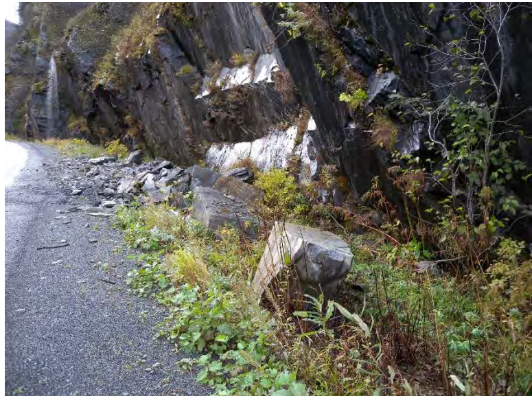
Rock slope at MP 18.12
