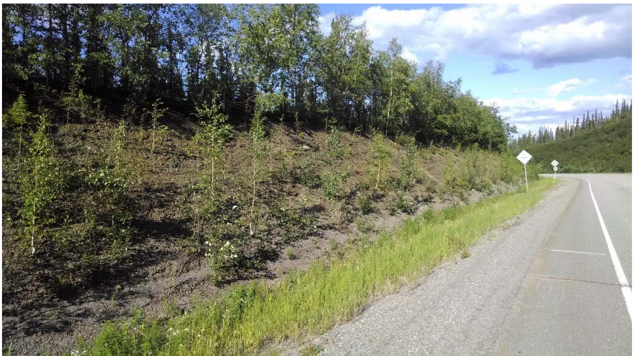
Figure 2-3: Class C rocky slope. Excluded from database due to stable configuration and short height. Either criteria would be sufficient. This could also be reasonably judged a soil slope due to the small rock size. Parks Hwy, approximately MP 340.
