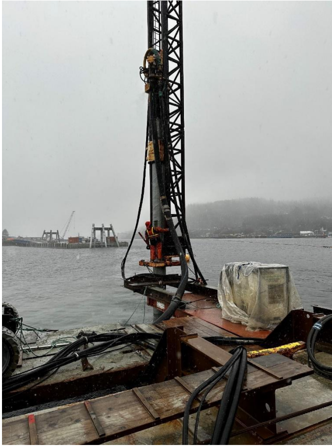
Figure 2. DTH drilling of a 24-inch diameter dolphin pile
