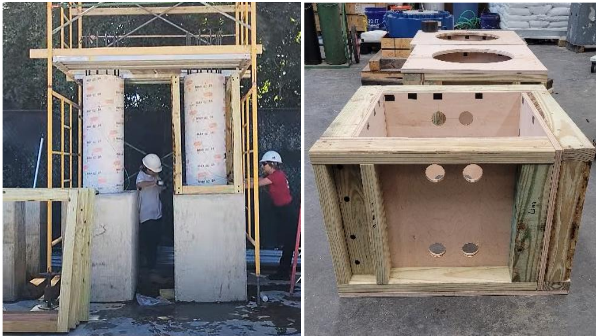
Figure 5-9 Formwork and frame support placement
