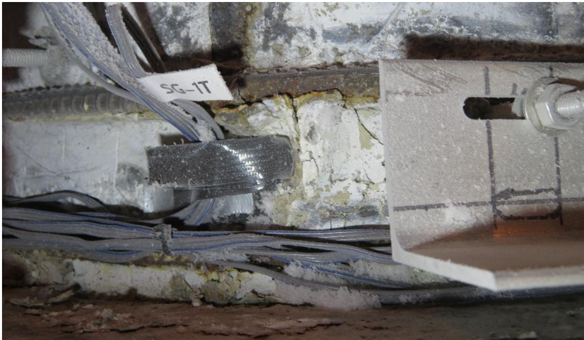
Figure 5-63 First cycle of \mu_4 (pulling). Initiation of concrete crushing
