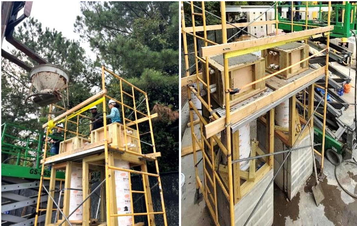
Figure 5-11 Column and cap beam concrete casting
