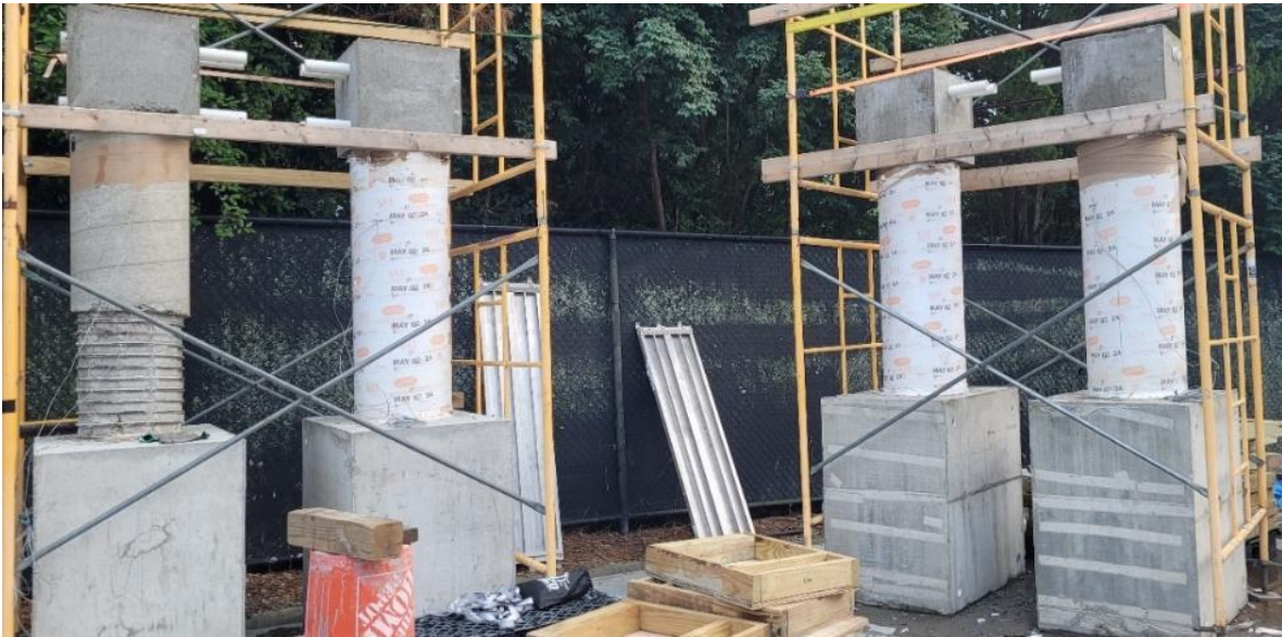
Figure 5-12 RC column specimens and removal of the formwork
