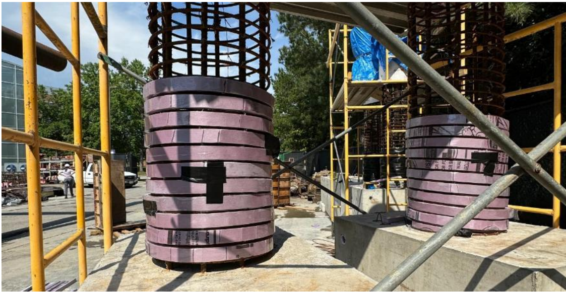
Figure 5-8 Foam blocks used to expose reinforcing steel along the plastic hinge.
