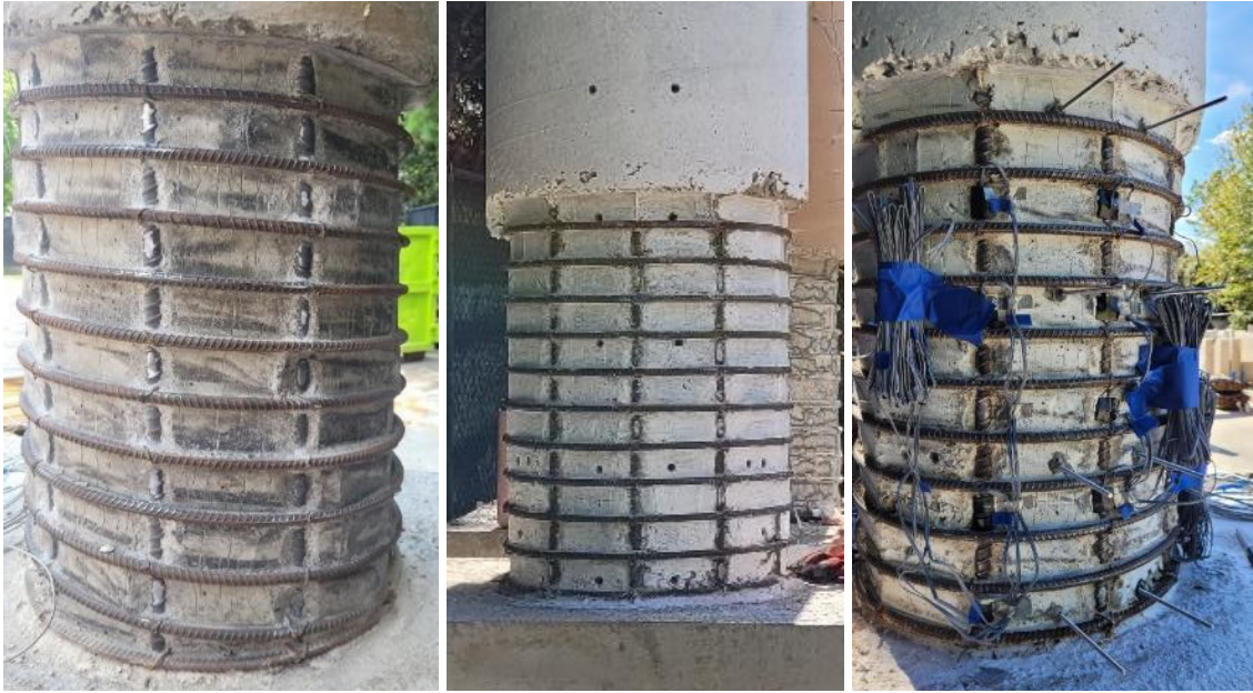
Figure 5-14 Cleaning of exposed reinforcing steel and column preparation for instrumentation
