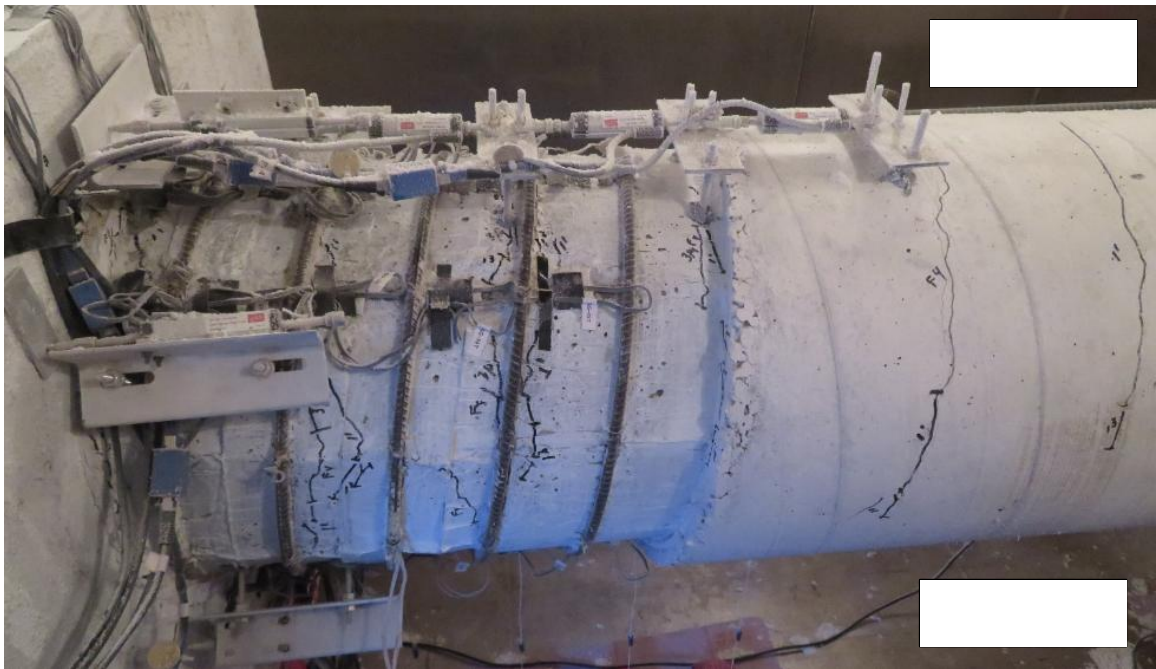
Figure 5-94 First cycle of \mu_1 (pushing): Extension of cracks
