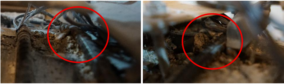
Figure 5-65 First cycle of \mu 5 : bar 2T buckled at the first pulling cycle and fractured in the subsequent pushing cycle
