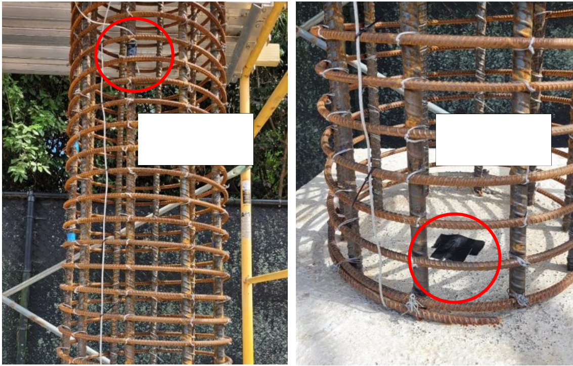
Figure 5-7 Thermocouples installation
