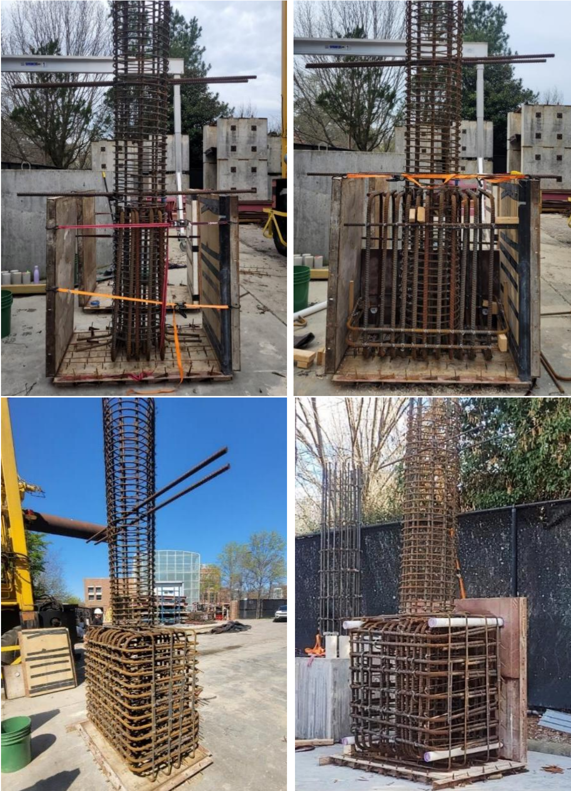
Figure 5-4 Footing cage construction and formwork
