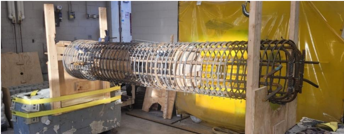
Figure 5-3 Column cage construction
