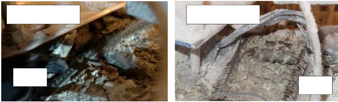
Figure 5-156 Top extreme bar buckling for the MA and QST columns with 2-inch spiral spacing tested at low temperatures.
