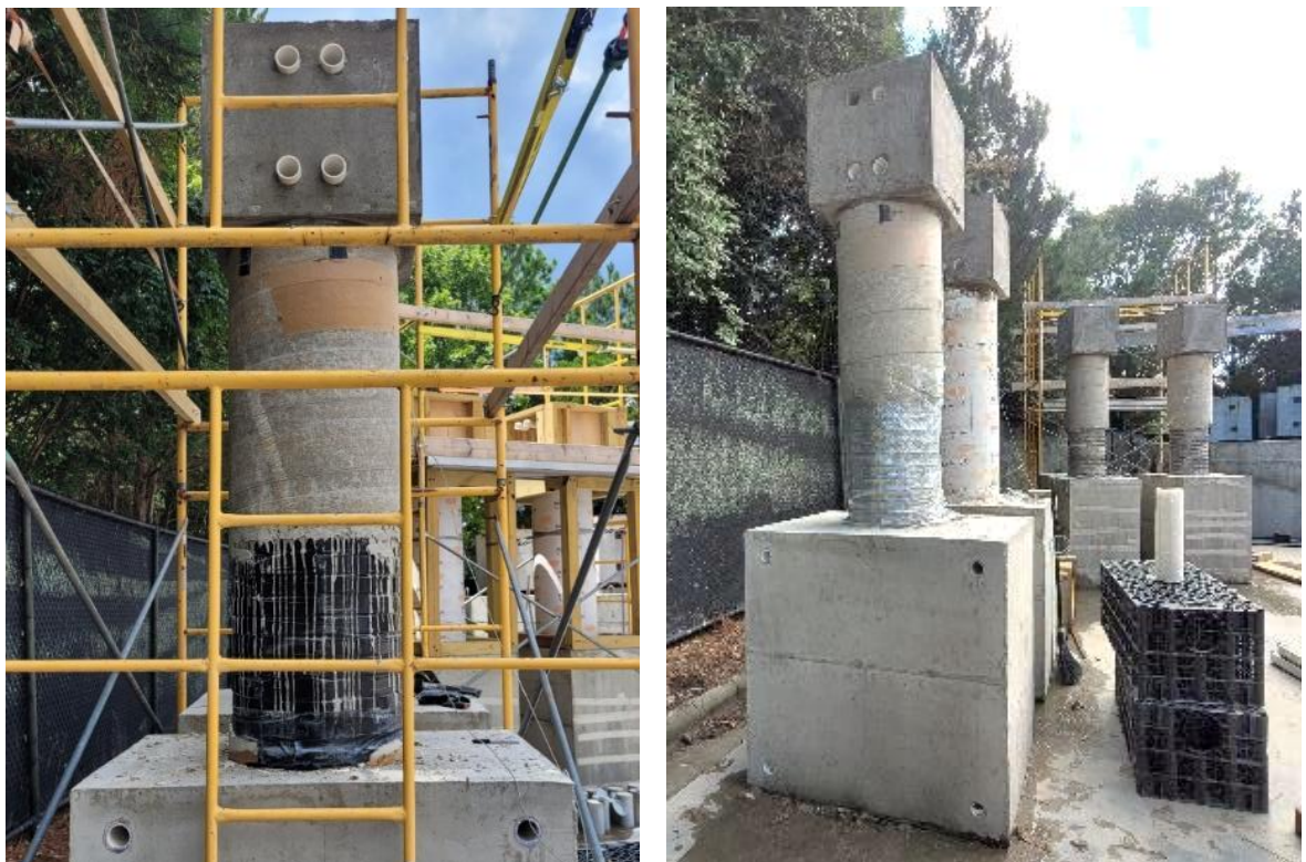
Figure 5-13 Removal of the formwork
