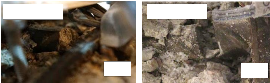
Figure 5-157 Top extreme bar fractures for the MA and QST columns with 2-inch spiral spacing tested at low temperatures
