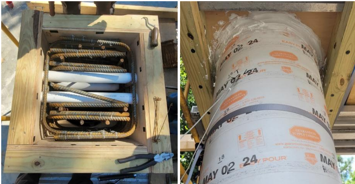
Figure 5-10 Placement and sealing of cap beam steel and PVC pipes, and placement of formwork
