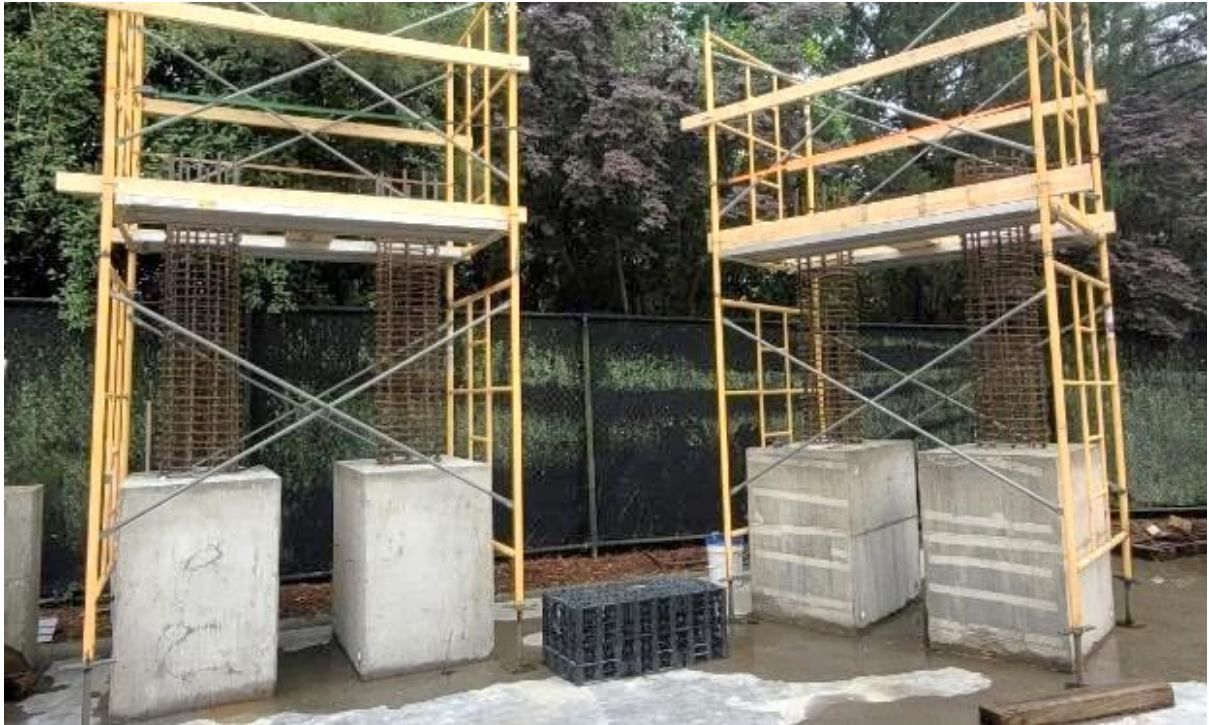
Figure 5-6 Placement of the specimens and scaffolding for column and cap beam construction
