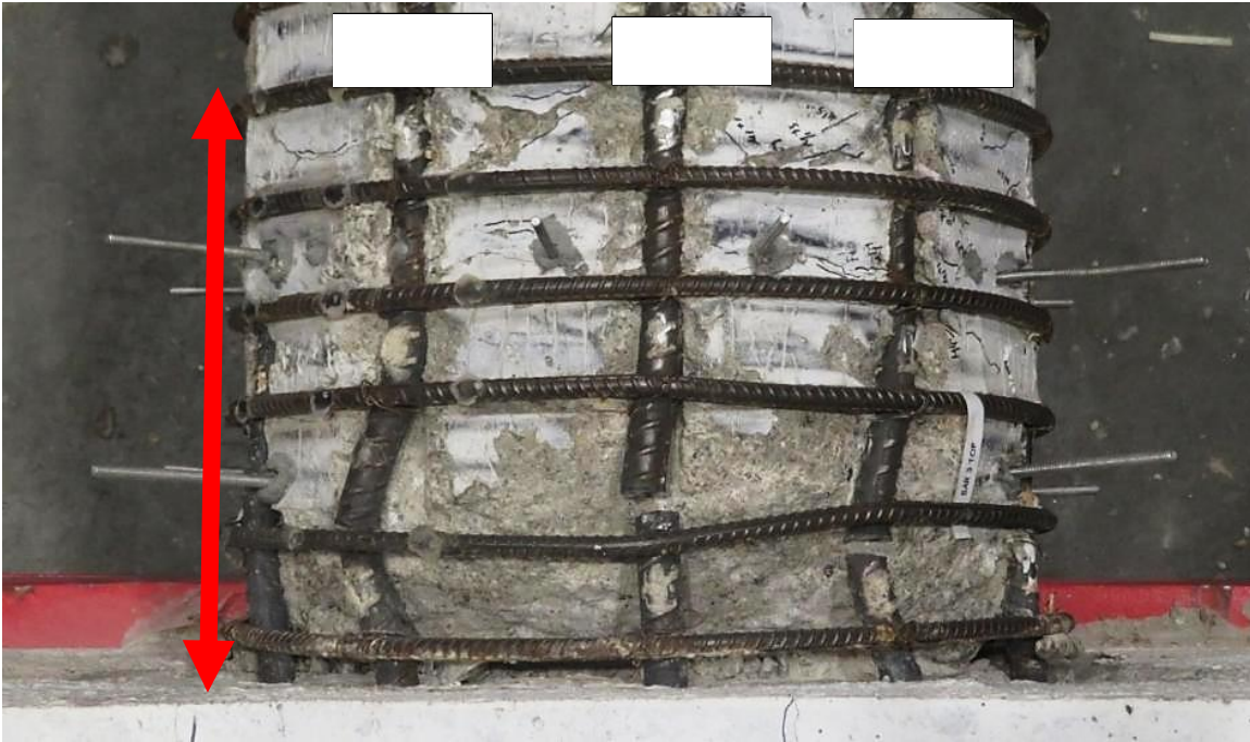
Figure 5-34 Final state of the specimen: Fracture of bars 1T, 2T, and 3T, and concrete core crushing.
