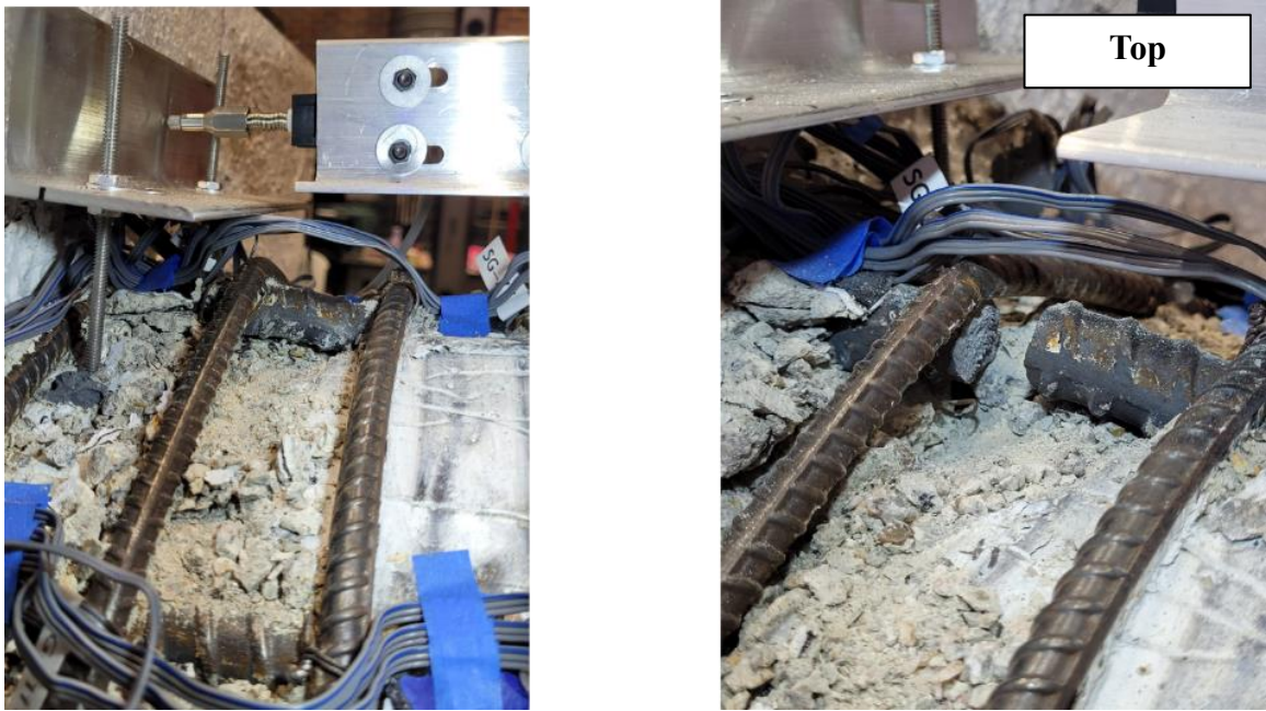
Figure 5-31 Third cycle \mu_5 : Visible bar buckling in pulling cycle and fractured in pushing cycle of the top extreme bar 2T
