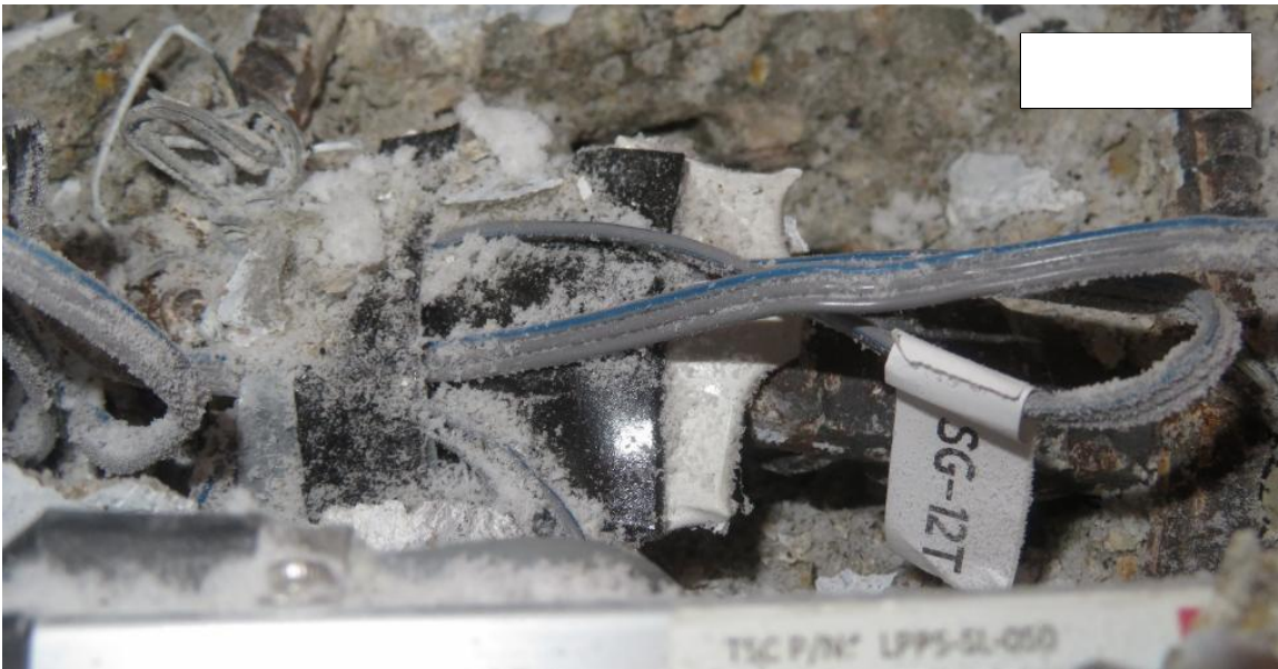
Figure 5-100 Third pulling cycle of \mu 5 : Visible buckling of adjacent bar to top bar, 3T
