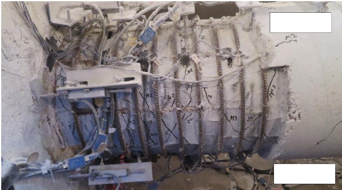
Figure 5-79 First cycle of \mu_3 (pushing) visible shear cracks and extension of existing cracks
