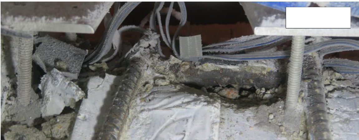
Figure 5-98 First pulling cycle of \mu 5 : Visible buckling of top extreme bar, 2T
