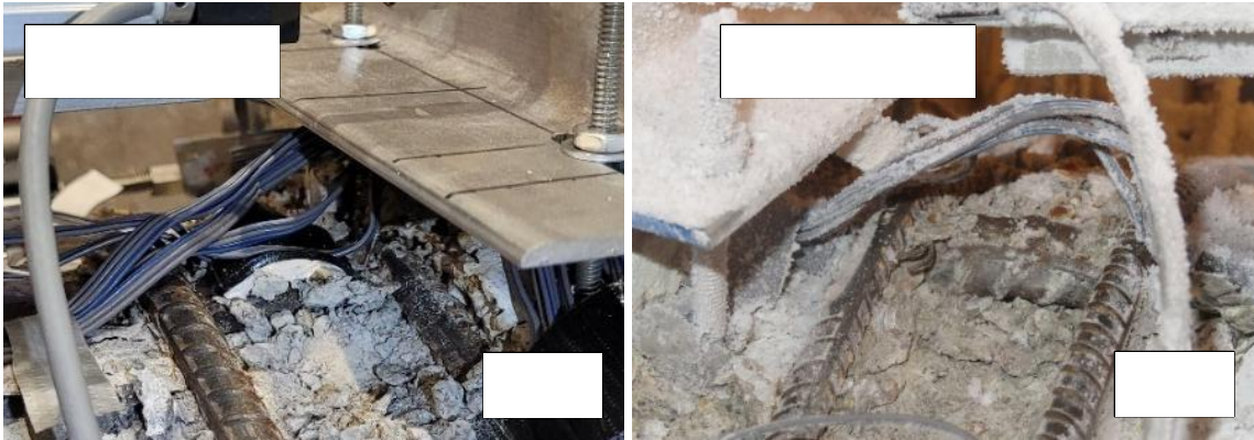
Figure 5-139 Buckling of the top extreme bar in the QST columns, tested at room and low temperatures.
