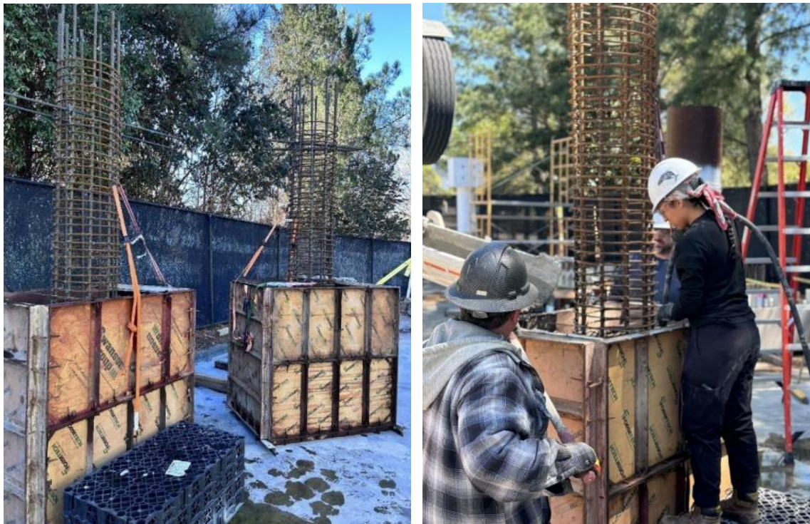
Figure 5-5 Footing's concrete casting
