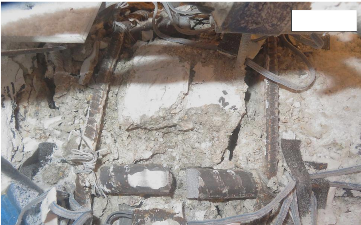
Figure 5-101 Third pushing cycle of \mu 5 : Bar fracture of bottom bar, 3B
