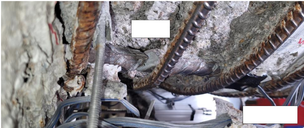
Figure 5-49 First cycle \mu_6 (pulling): buckling of top bar 3T, and fracture of bottom extreme bar 2B
