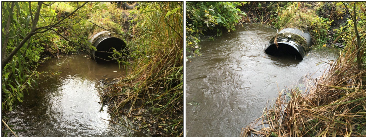
Figure 5.—Egan Drive Creek culvert inlet; low flow 9/20/2023 (left), high flow 9/21/2023 (right).
