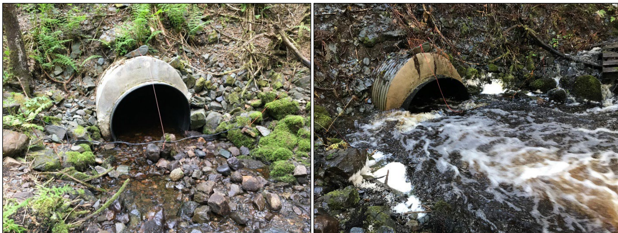
Figure 3.—Ninemile Creek culvert inlet with PIT tag antenna installed; low flow 5/28/2023 (left), high flow 10/19/2023 (right).
