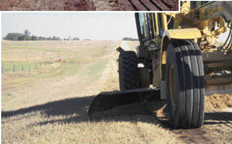
The material from the high shoulder is then pulled into the cut that has just been made. Generally, this material will have to be worked several times with the grader to break it up enough to spread evenly.
