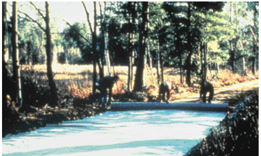
A decision was made to stabilize the above road. A road crew is shown rolling out a fabric over the existing road surface.
