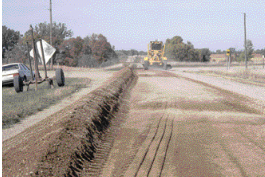
The motorgrader operator has done a good job of picking up the fresh gravel and equalizing it into a very uniform windrow.
