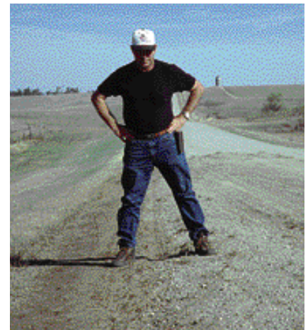
The windrowed gravel is then brought back over the recovered material and the roadway is restored to proper crown and shape. The high shoulder has been eliminated.
