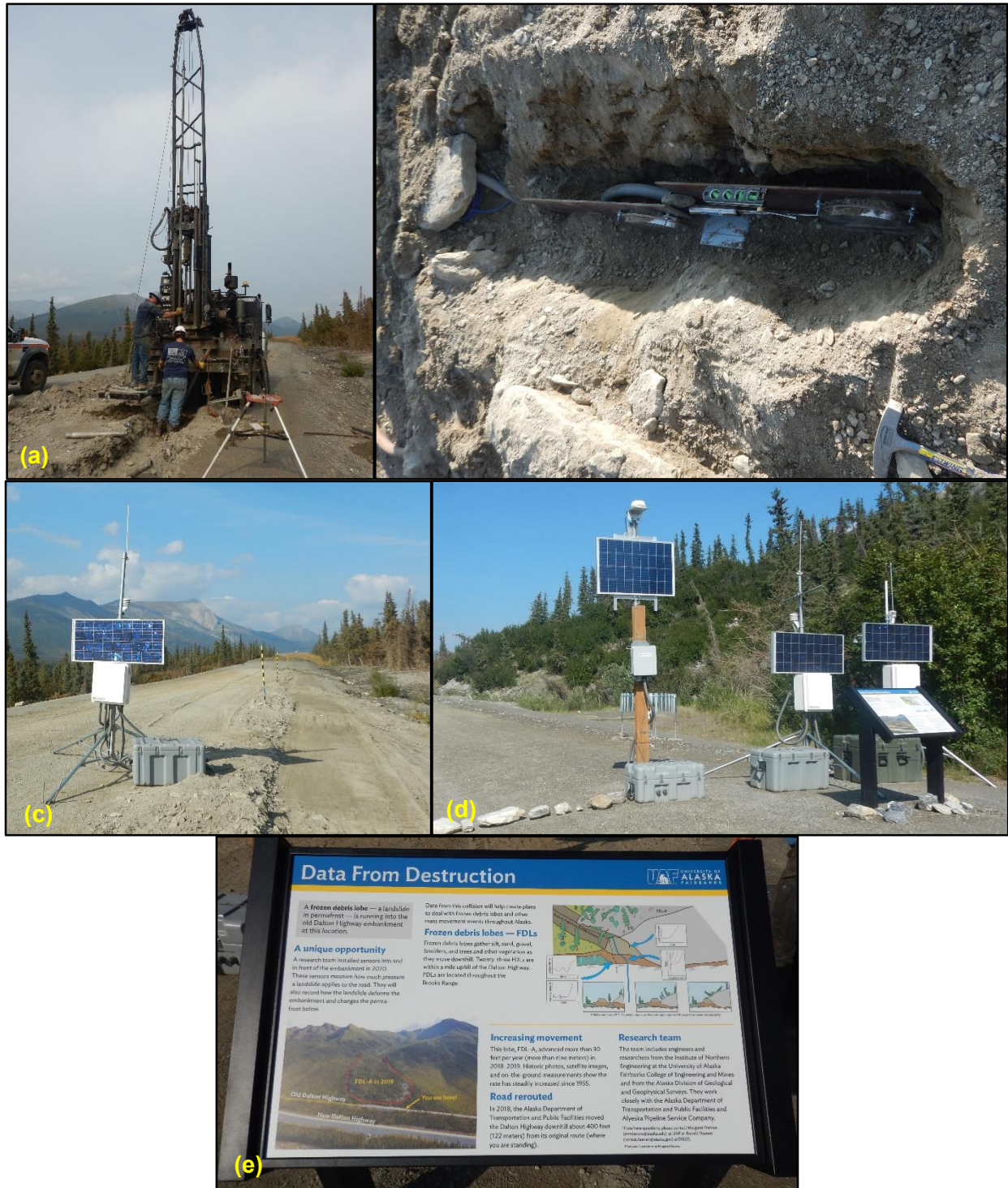
Figure 2. Images from the 2020 drilling program: a) drill truck centered on trench to drill TH20-03; b) looking down at the pressure plates and tilt meter embedded into the uphill side slope of the embankment near TH20-02; c) looking to the north at the 2020 location of the secondary ADAS moved to accommodate the short cables; d) all ADAS at the southern end of the project location in 2022; e) interpretative display installed as an outreach component.
