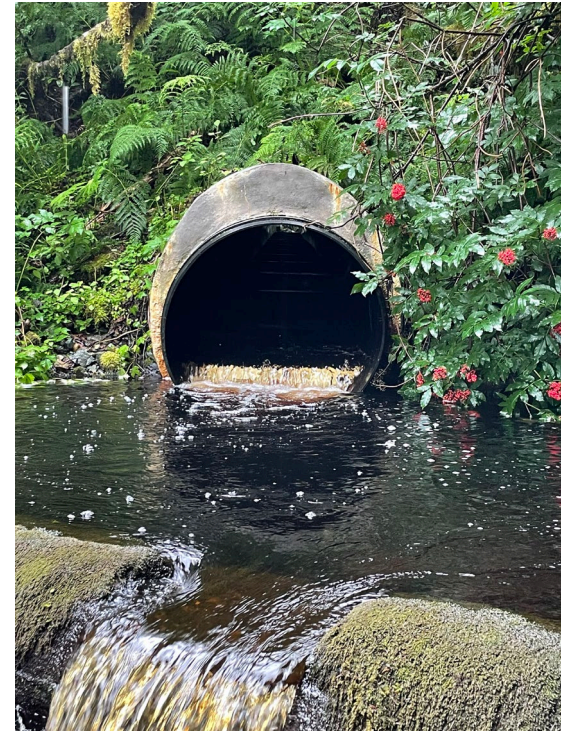
Slip lined culvert at 9-mile Creek in Juneau, AK where fish pass trials were conducted.
