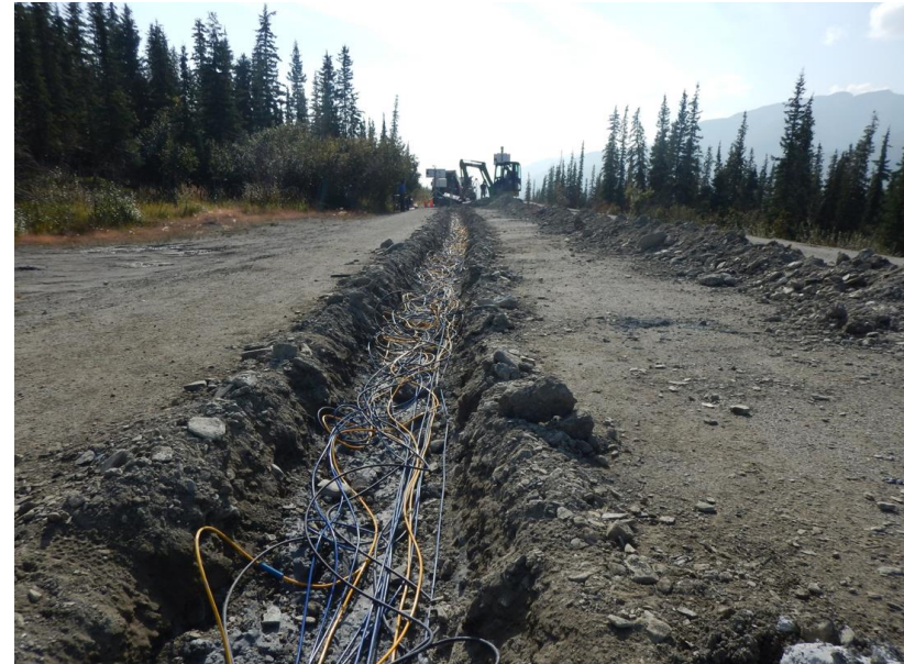
Installing sensor equipment- Dalton Highway- Shane Moller, DOT&PF
