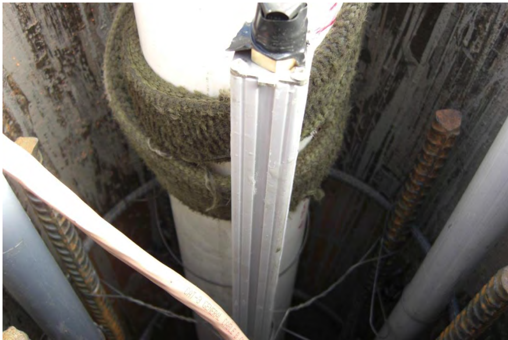
Figure 2.7: Inclinator as installed in the test pile.
