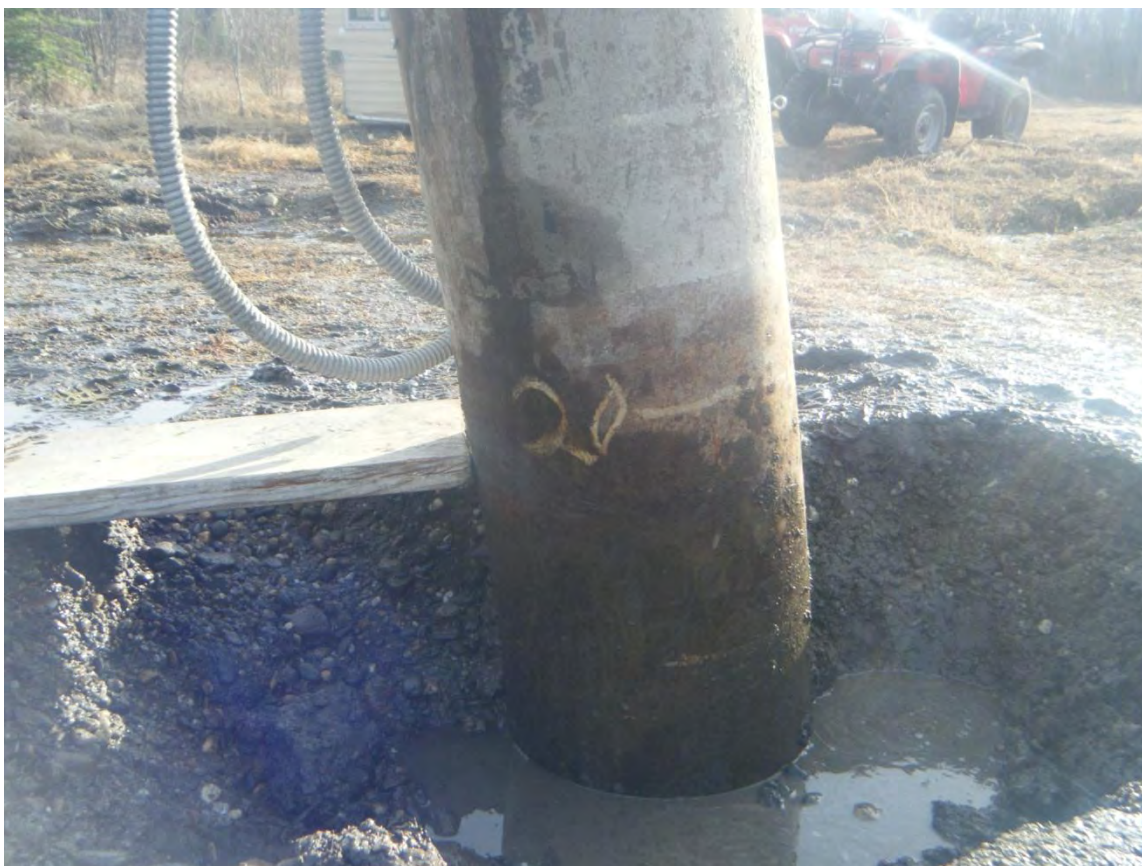
Figure 2.54: Excavation of south pile tested March 2010.
