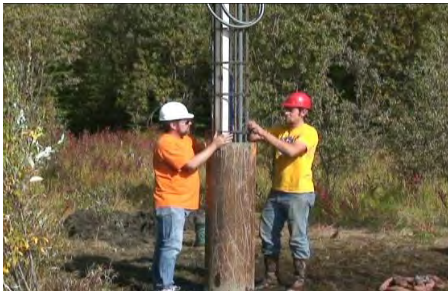
Figure 2.10: Installing a reinforcing steel cage with sensors into a test pile (photo by INE staff).
