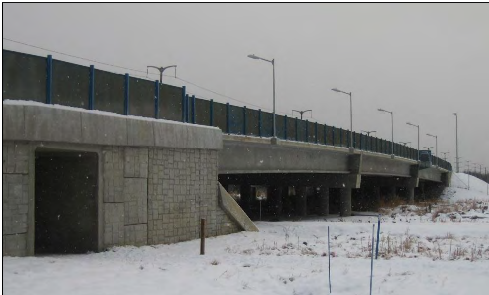
Figure 3.3: North Fork Campbell Creek Bridge.
