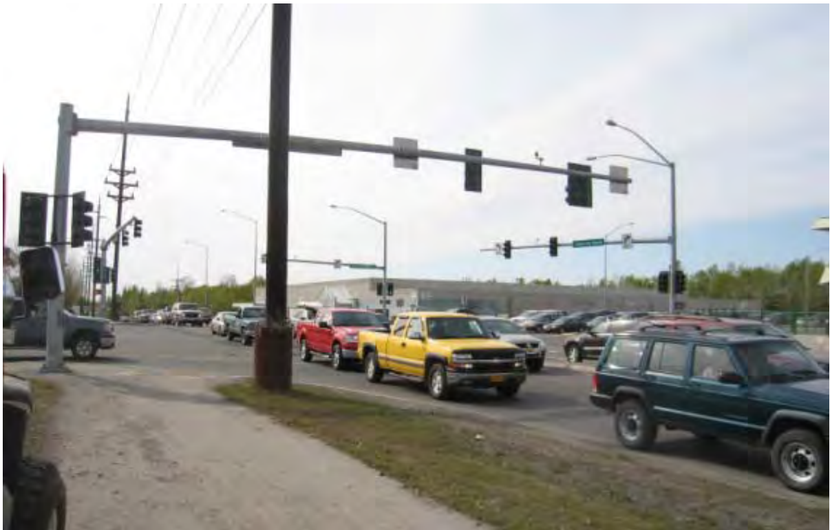
Figure 3 Picture showing the queue from the eastbound entrance approach blocking the upstream intersection at Old Seward Highway/E. Dowling Road
