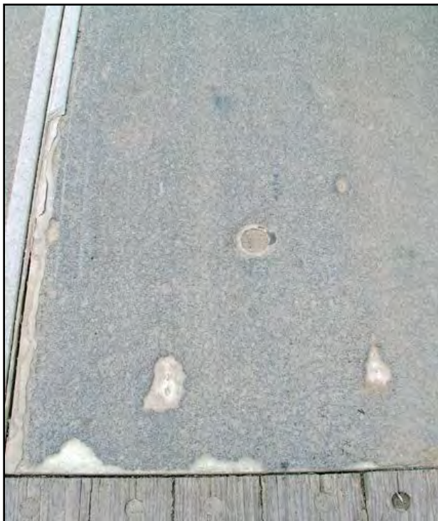
Figure C.7 Transonite panel, 2007 (2 years old).
