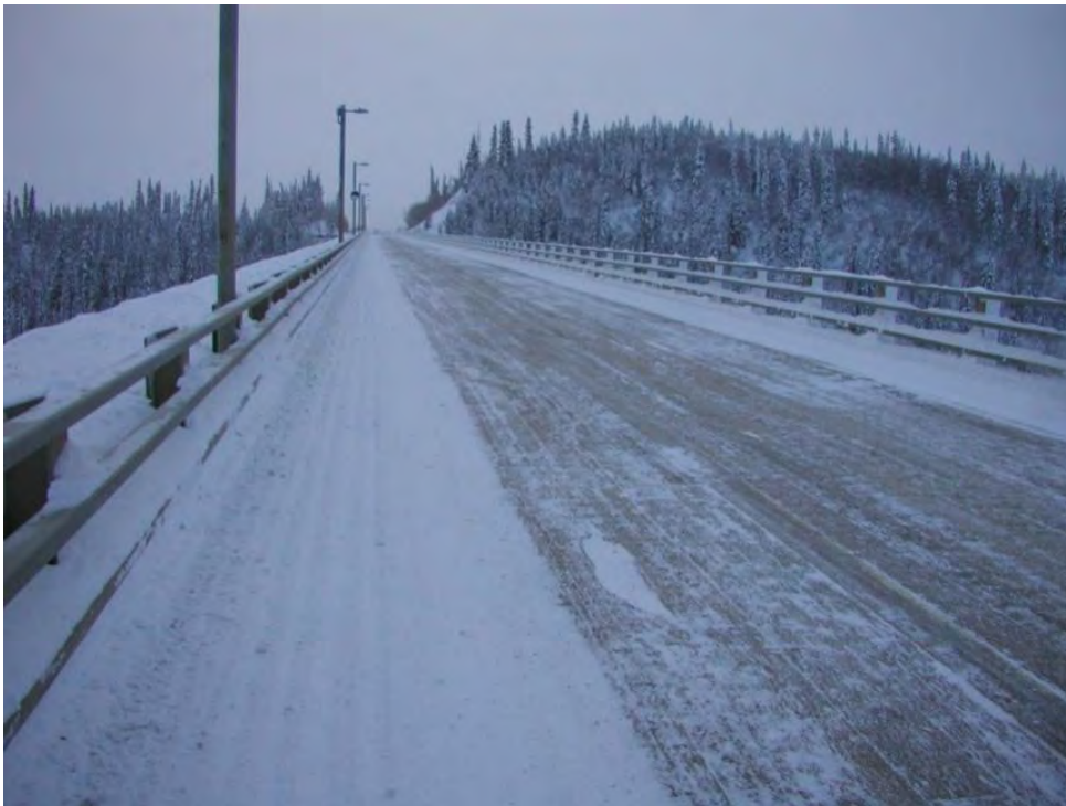
Figure 2.2 Yukon River Bridge in winter looking up the 6% grade.
