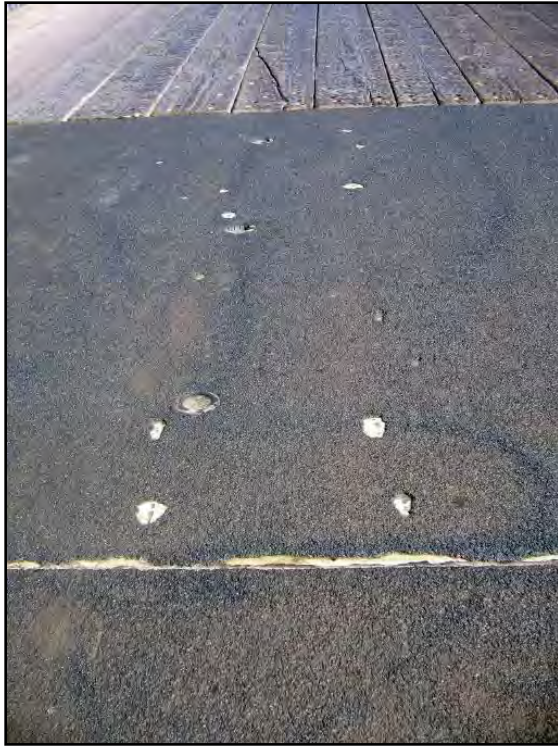
Figure C.6 Transonite panel, 2006 (1 year old).
