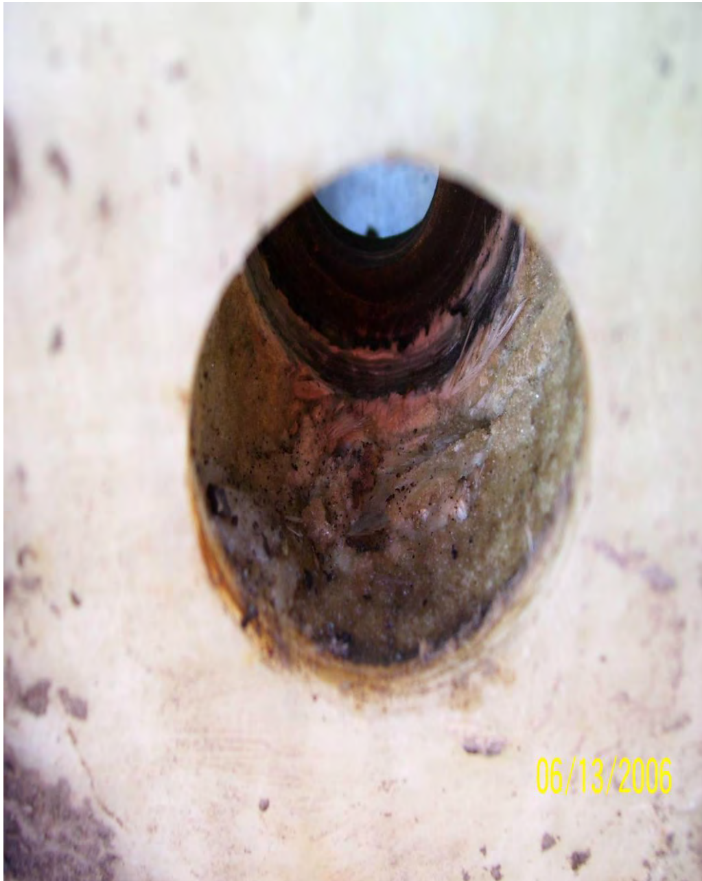
Figure B.18 Hole for the insert: looking from the bottom.
