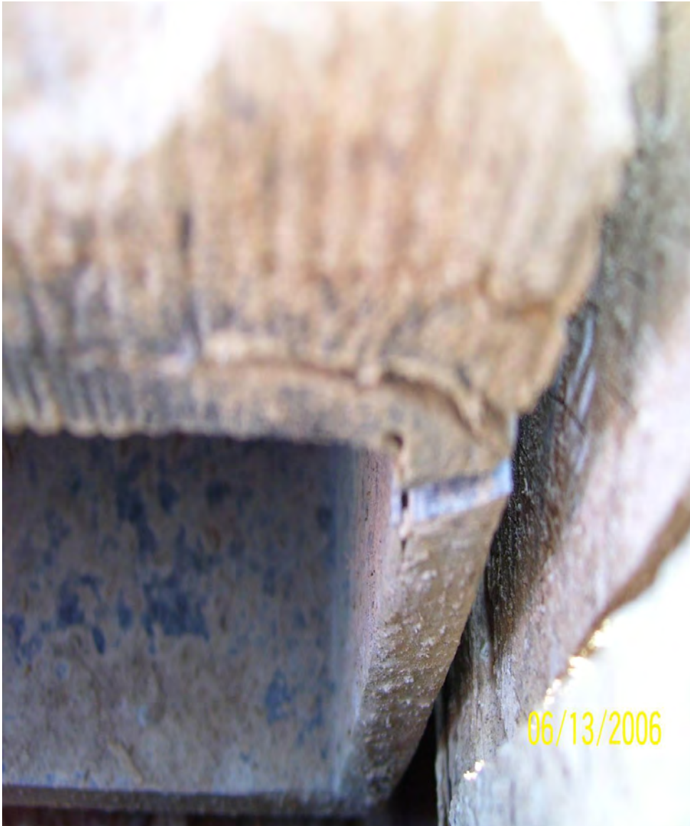
Figure B.24 Prodeck 4 test panel: Cracked fiberglass end.
