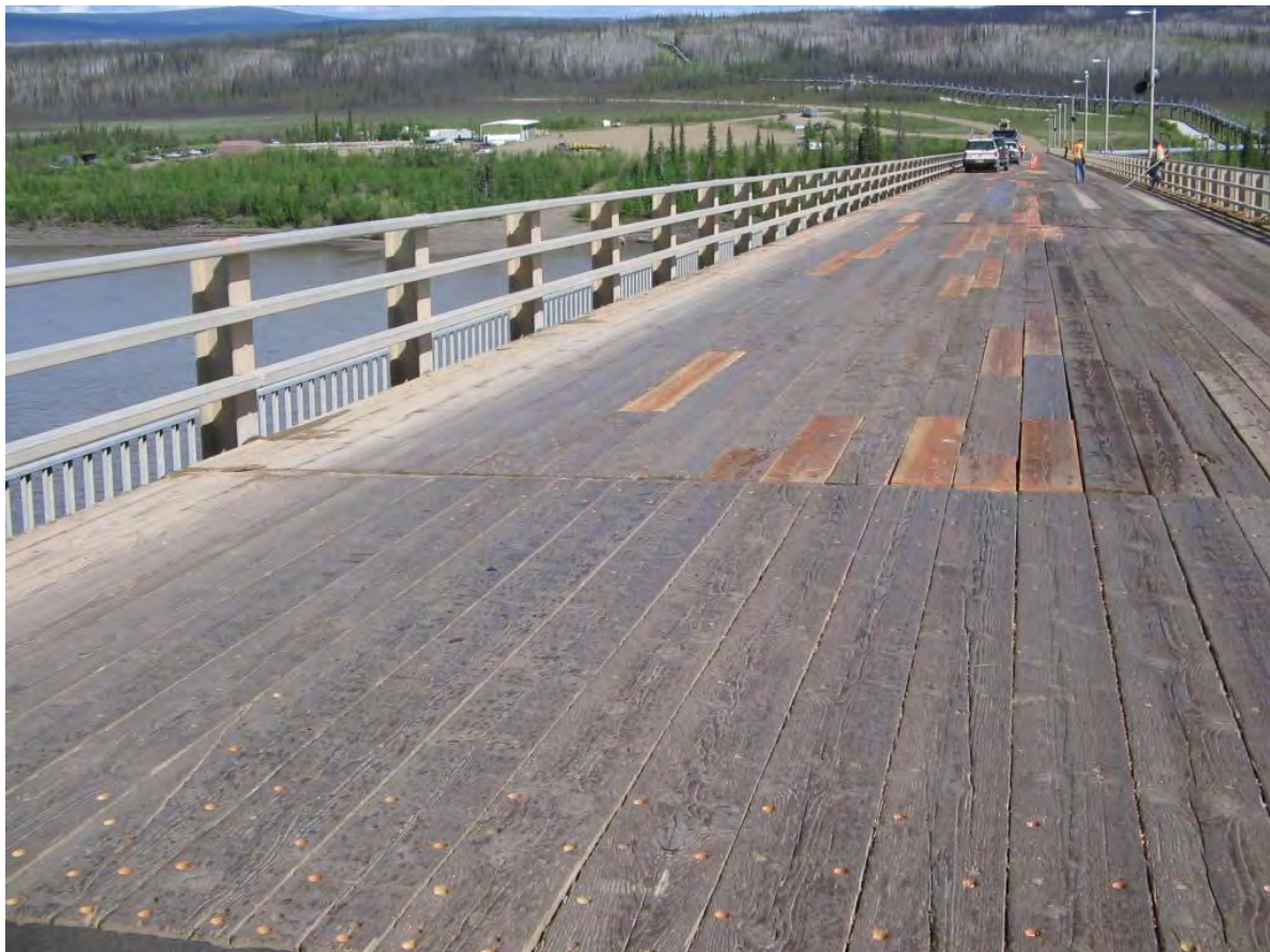
Figure 1.1 Timber deck repair, a maintenance activity.
