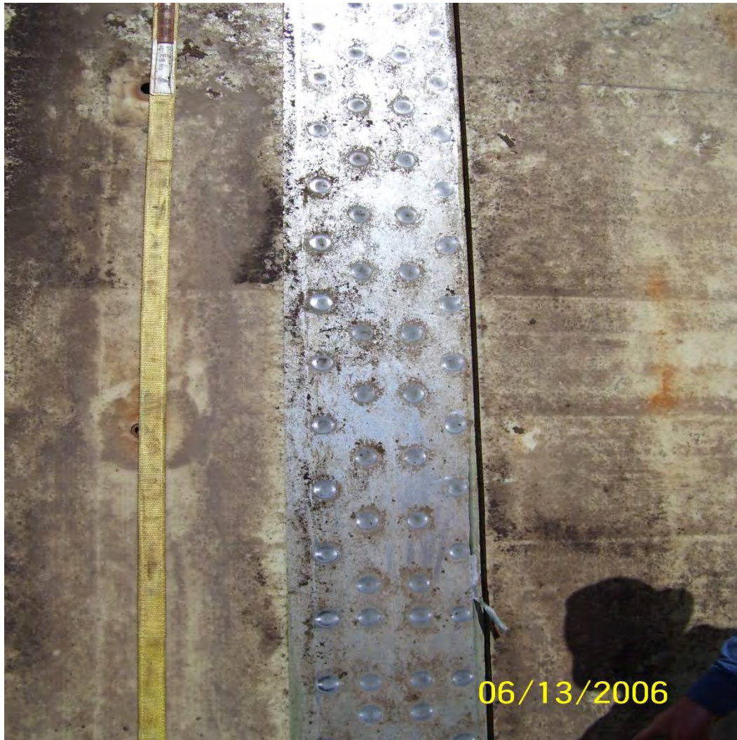
Figure B.19 Bolted splice plate supporting deck panels
