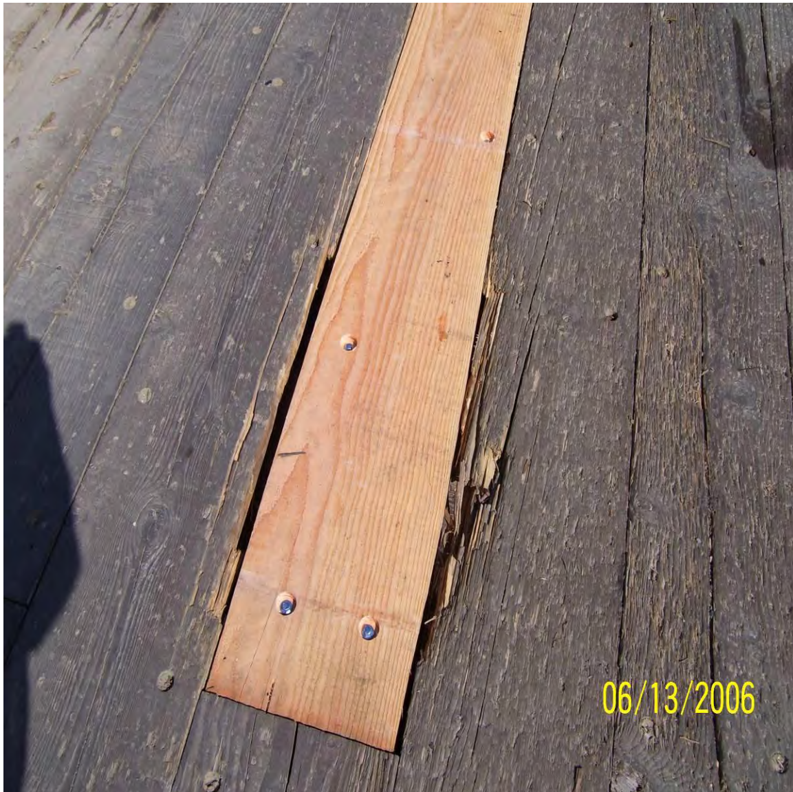
Figure B.5 Wood wearing surface: A typical replacement by Maintenance.
