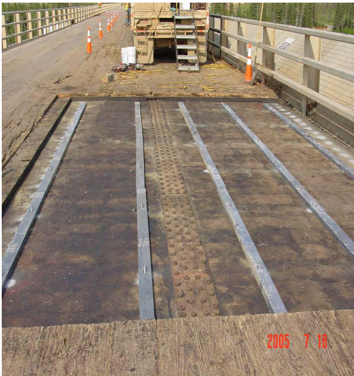
Figure B.25 Installation of Prodeck 4 on the Yukon River Bridge (after AKDOT&PF).
