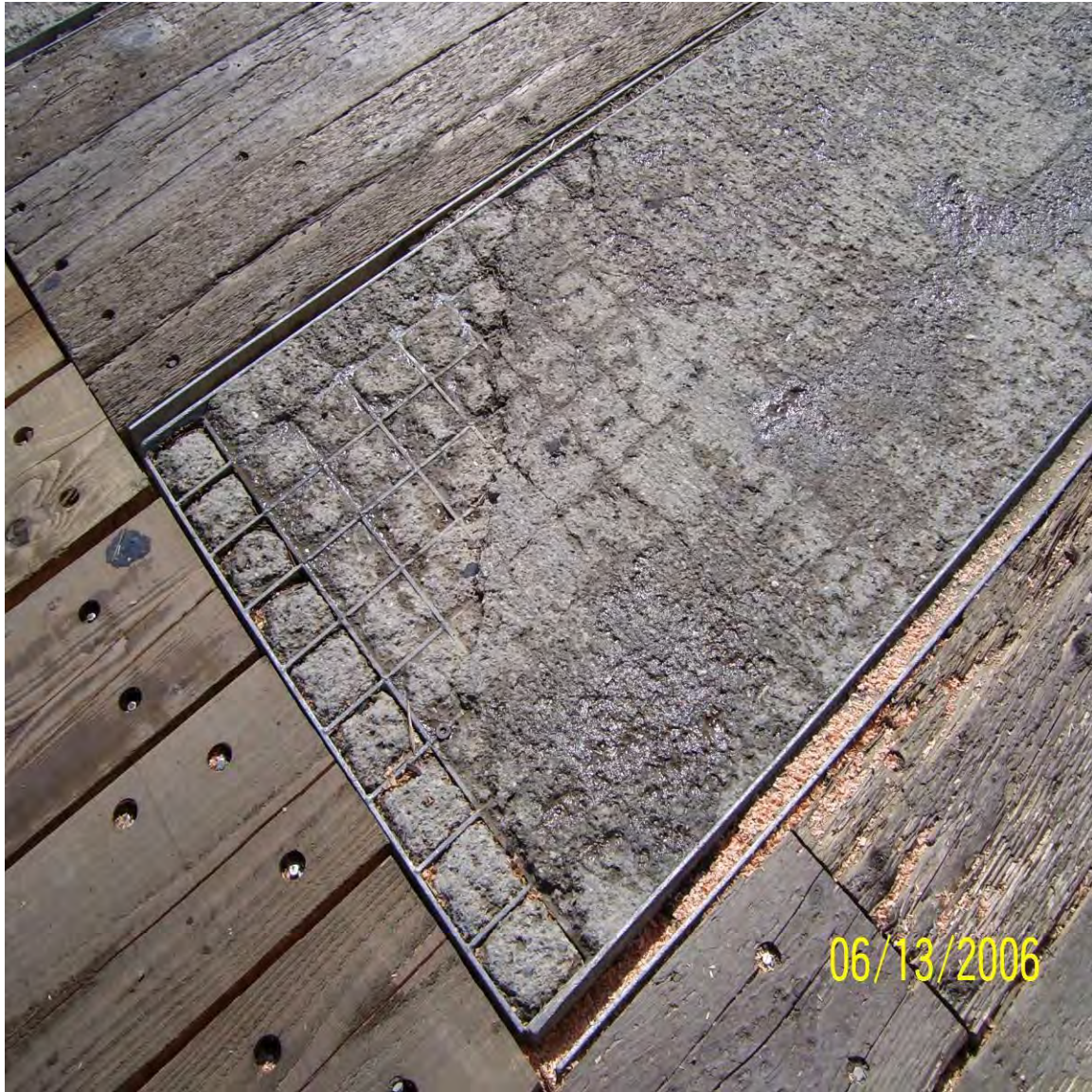
Figure B.6 Concrete-filled steel grid wearing surface (7 years old).
