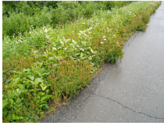
Photo 11. Desirable and undesirable vegetation intermixed in zones 1 and 2
