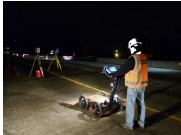
(b) Use of GPR to Collect Data from Concrete Bridge Deck (Tarussov et al., 2013)
