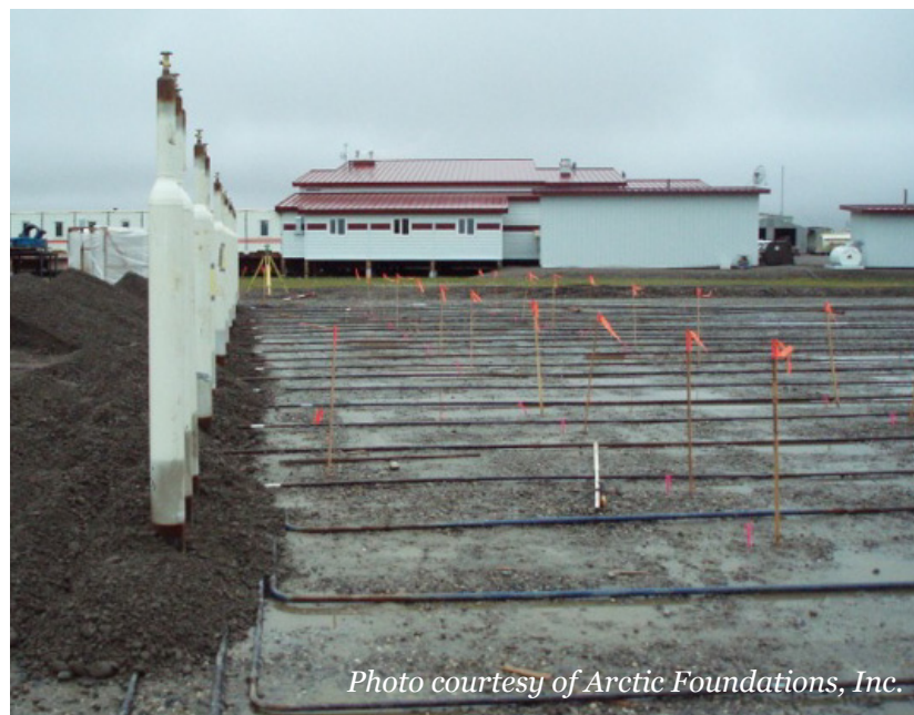
b. Thermosyphons prior to fin installation.
