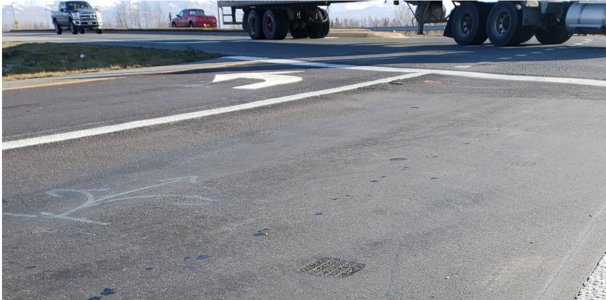
Photo 9 - Ramp 6 Deformation
