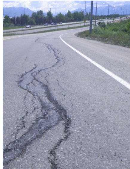
Photo 2 – Ramp 1 After Surface Preparation
