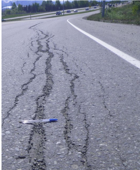
Photo 1 – Ramp 1 Prior to Surface Preparation
