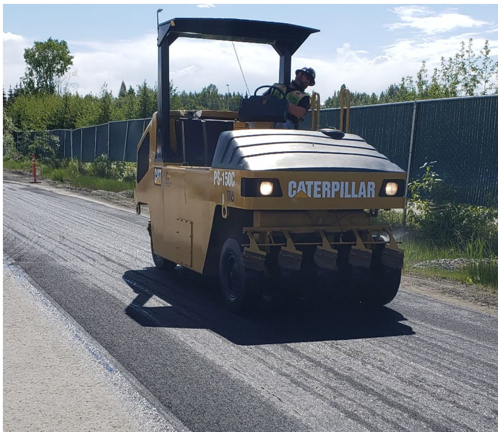
Photo 41 - Pneumatic Roller on Test Strip
