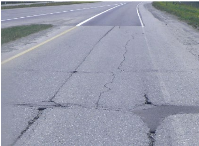
Photo 5 - Ramp 11 Prior to Surface Preparation
