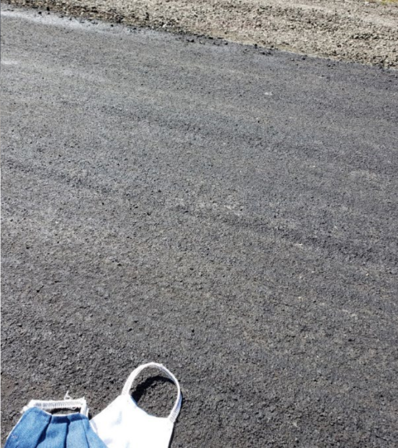
A mask on the microsurfacing test strip after the roller has made its passes and it has set.
