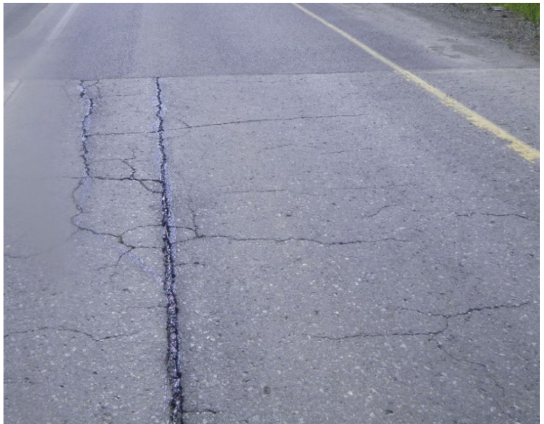
Photo 4 - Ramp 9 General Condition
