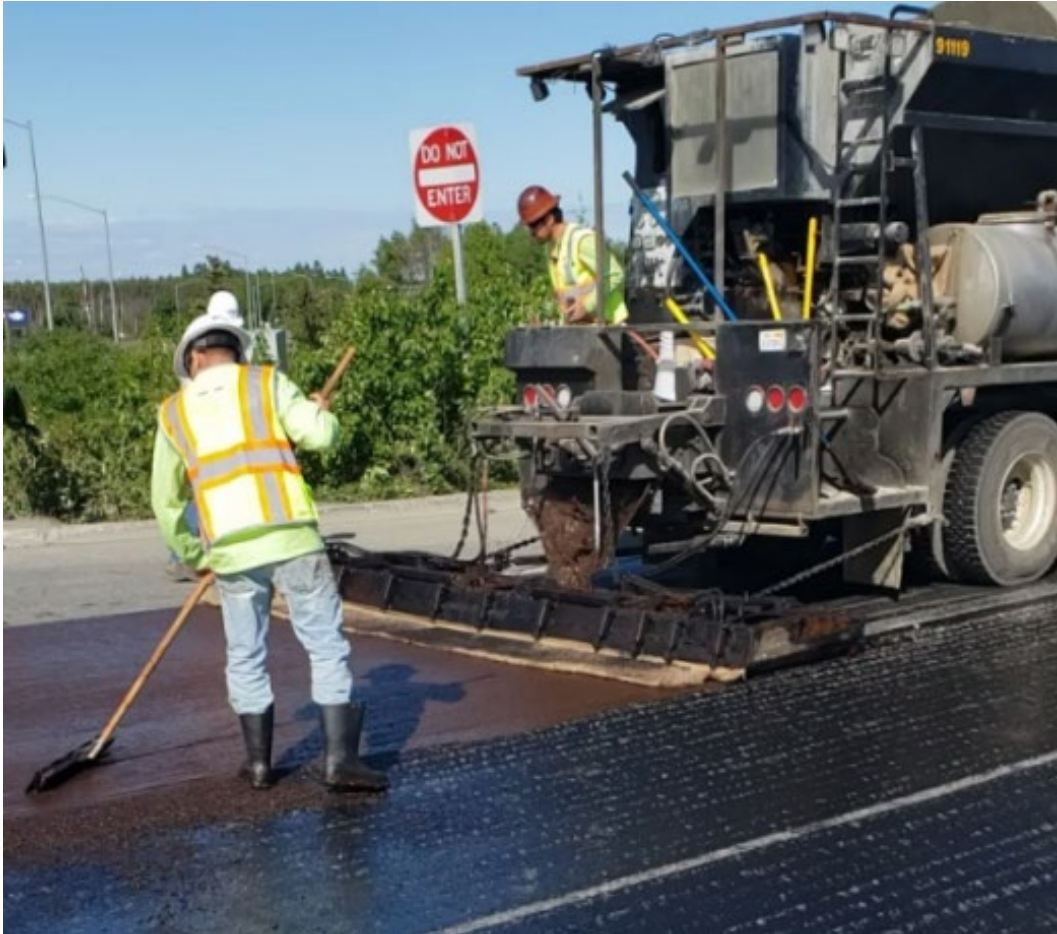
Scratch course placed on Ramp 5 prior to stopping production.
