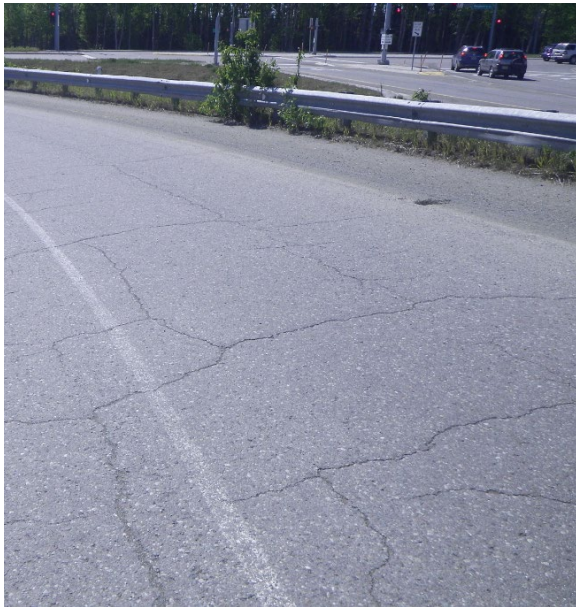
Photo 3 - Ramp 8 General Condition
