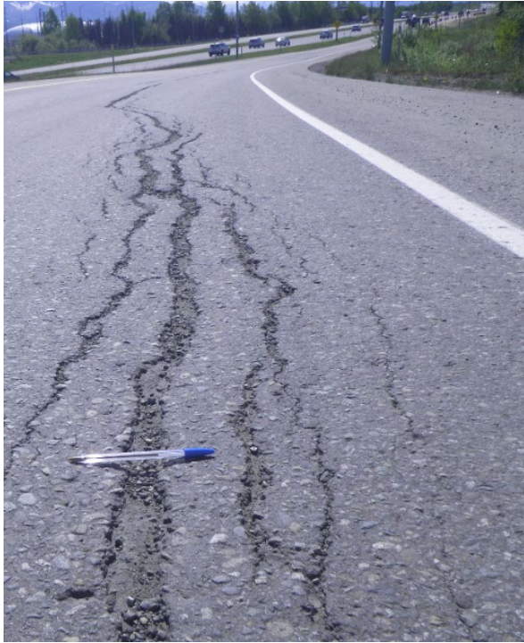
Ramp 1 Prior to Surface Preparation
