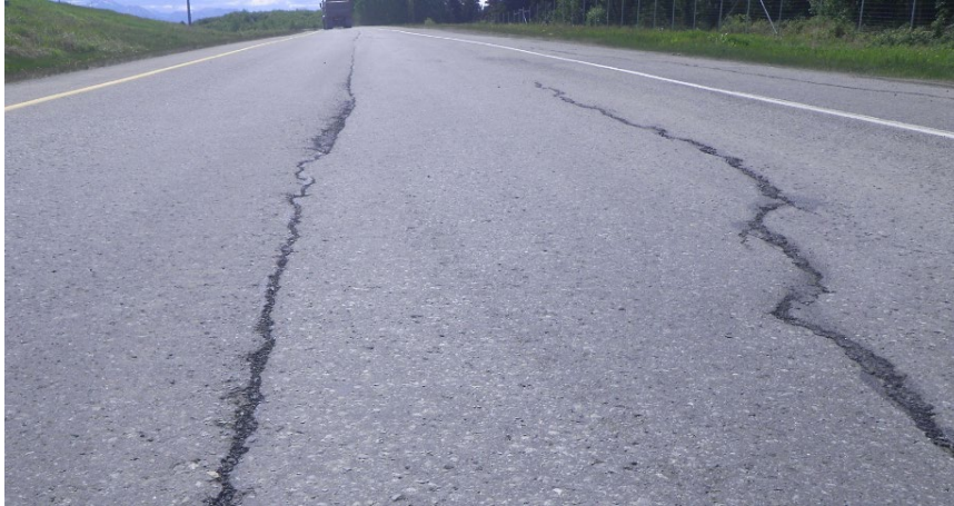
Photo 7 - Ramp 15 After Surface Preparation
