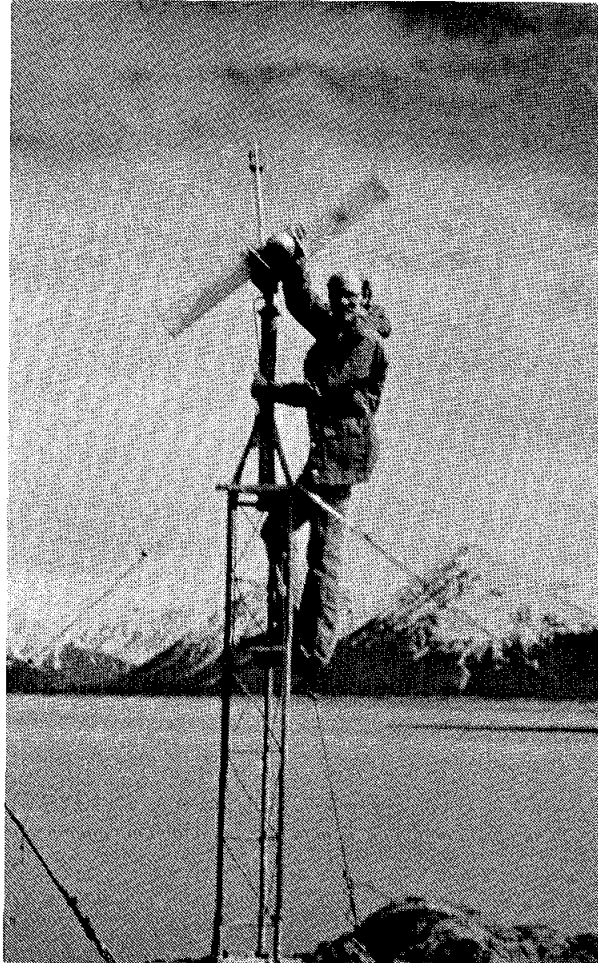
Figure 2 - 2: Lack of adequate tower height can cause severe turbulence
