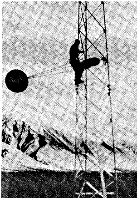
Fig. 4-6: Attaching generator to tower using gin pole. (Source: 4 Winds of Alaska)
