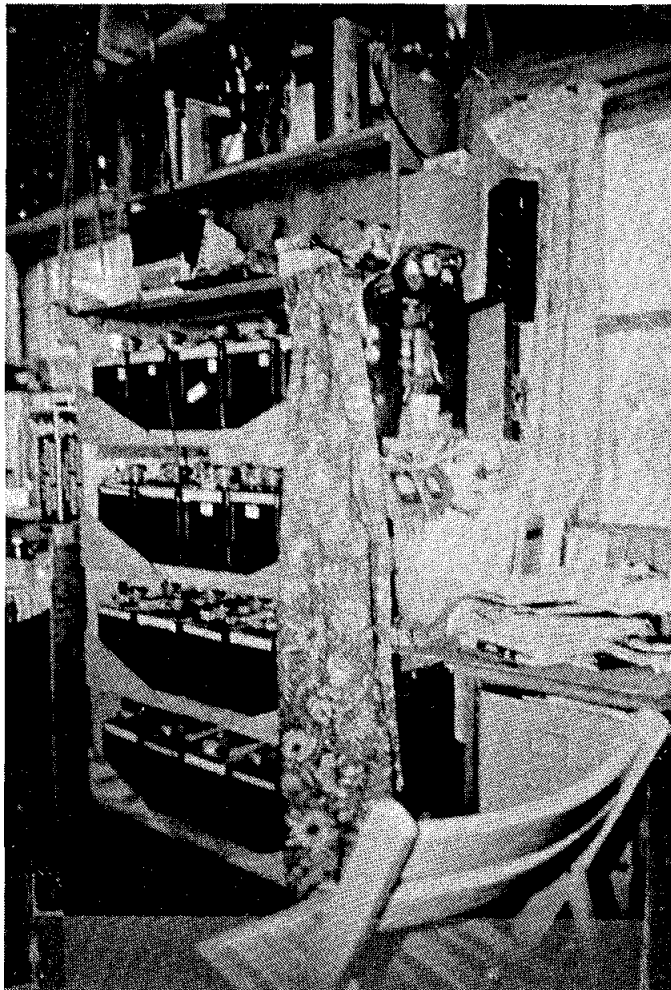
Figure 2 - 5: Batteries stored in living space in system built in the Arctic Region (Source: Newell)
