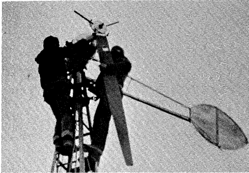
Fig. 4-7: Installing blades on windgenerator. (Source: 4 Winds of Alaska)
