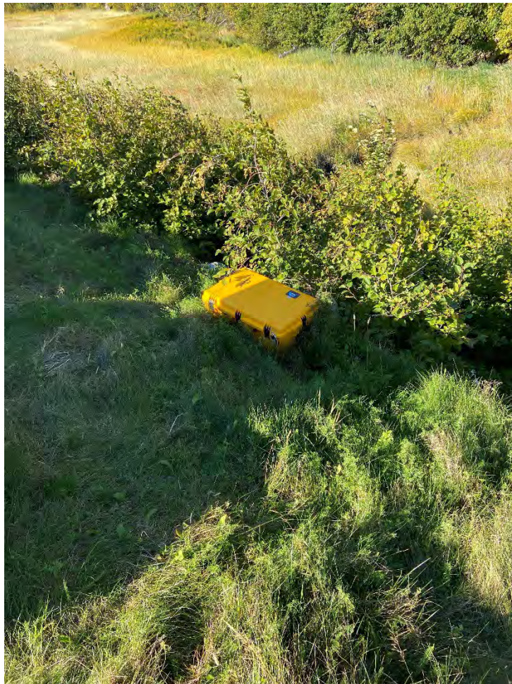
Seward Highway MP 98.5 battery box located on grassy hill north of station.
