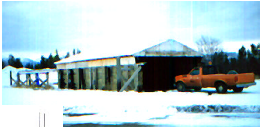
Above and left: Photographs of the Yukon salt sheds already in use. The roof opens to allow easy access to the salt stored inside. The roof is on tracks that permit it to roll backward with a slight push.
