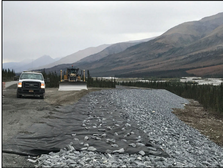
Figure 4: Geotextile Placed on top of ACE Shoulder.
