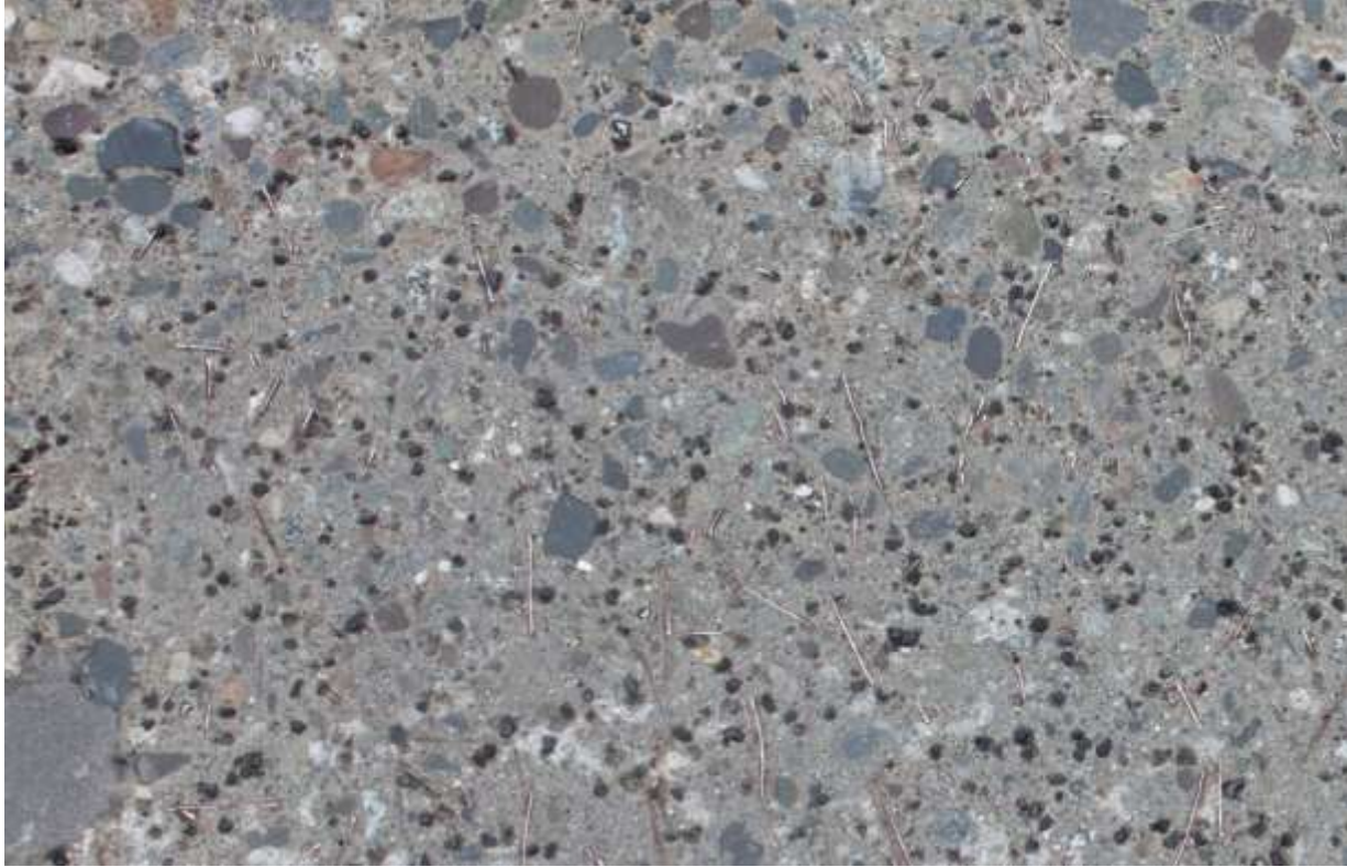
Figure 19: Steel fiber in the test section (Abaza, July 2020).
