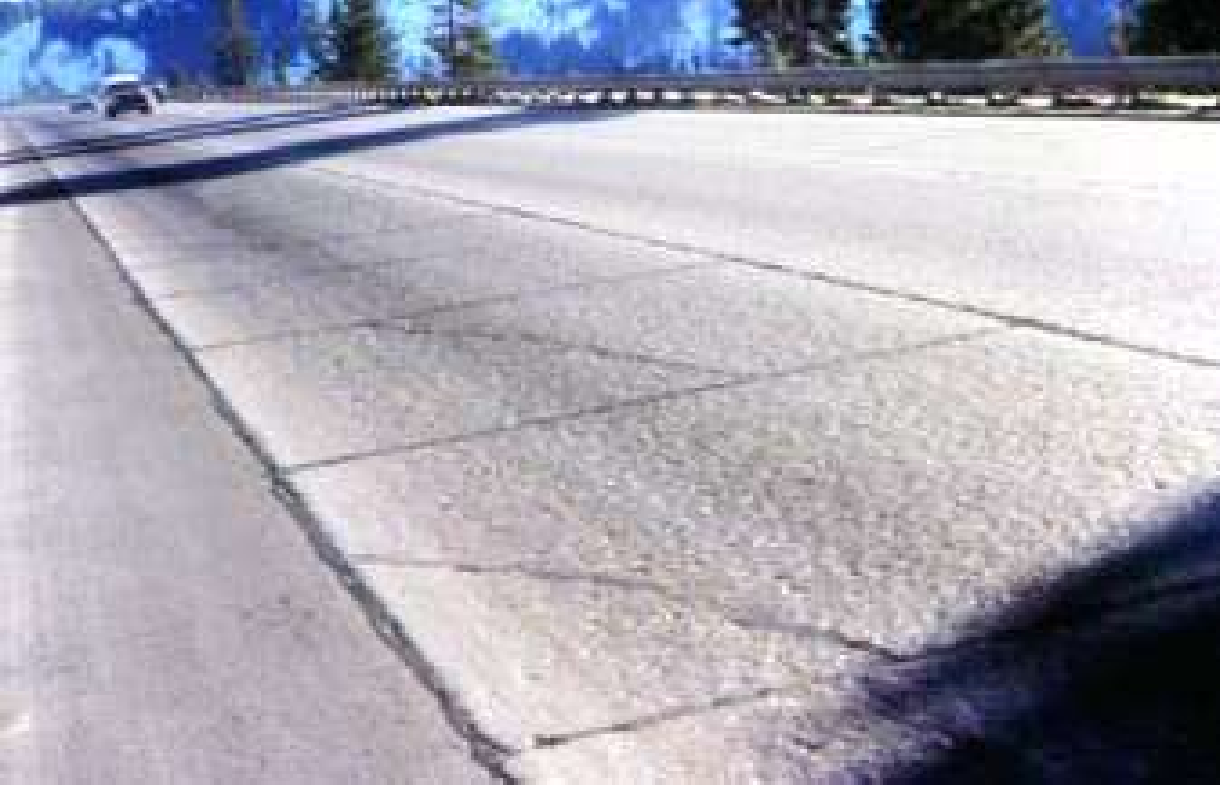
Figure 15: Typical rigid pavement rut (PCA [70156]).
