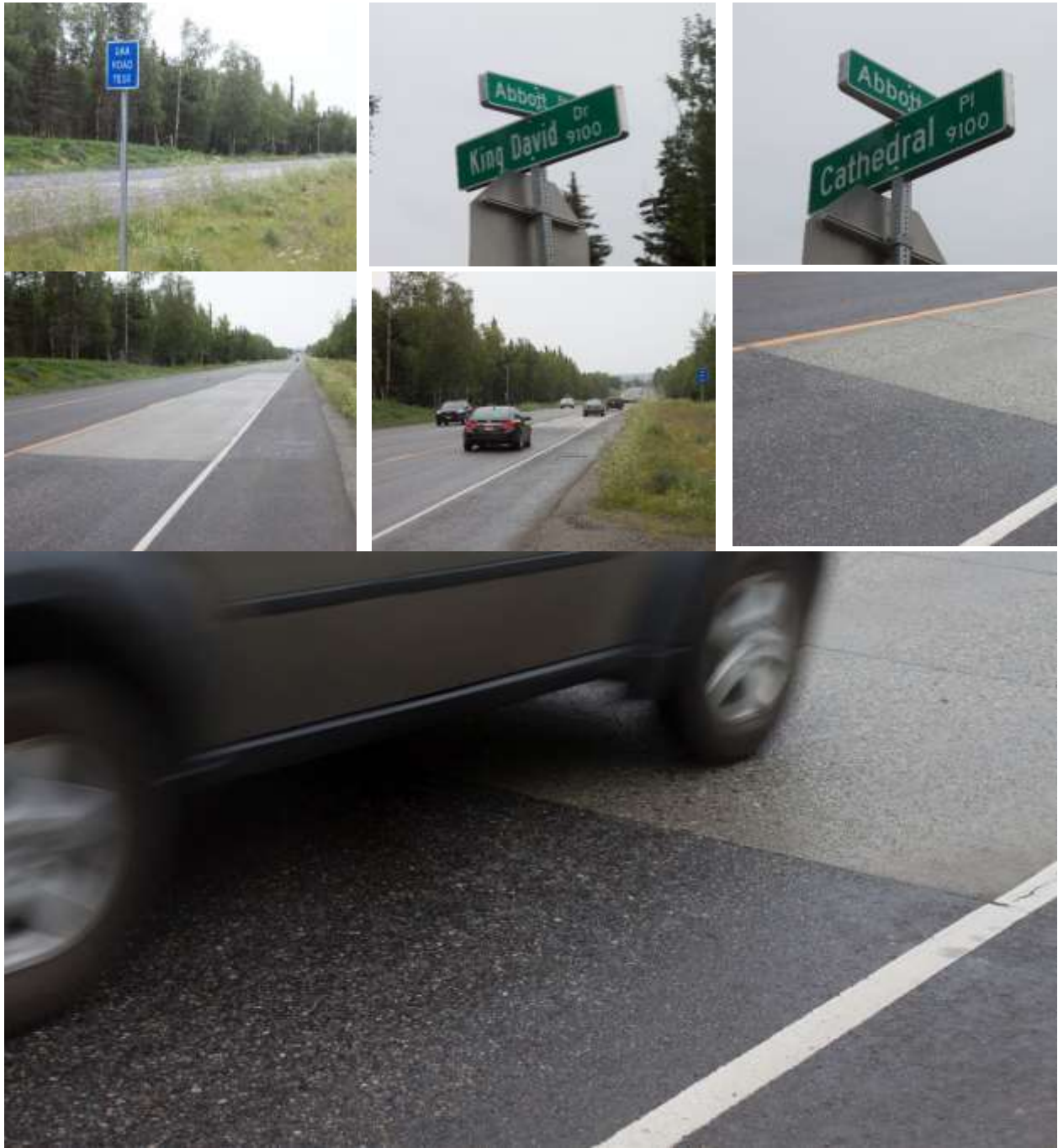
Figure E10: Snapshots of the SFRRRC test section and HMA after about 3 years of service.
