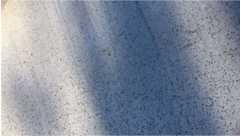
Figure 7: Typical close-up view of the SFRRRC surface (Abaza, 2018).
