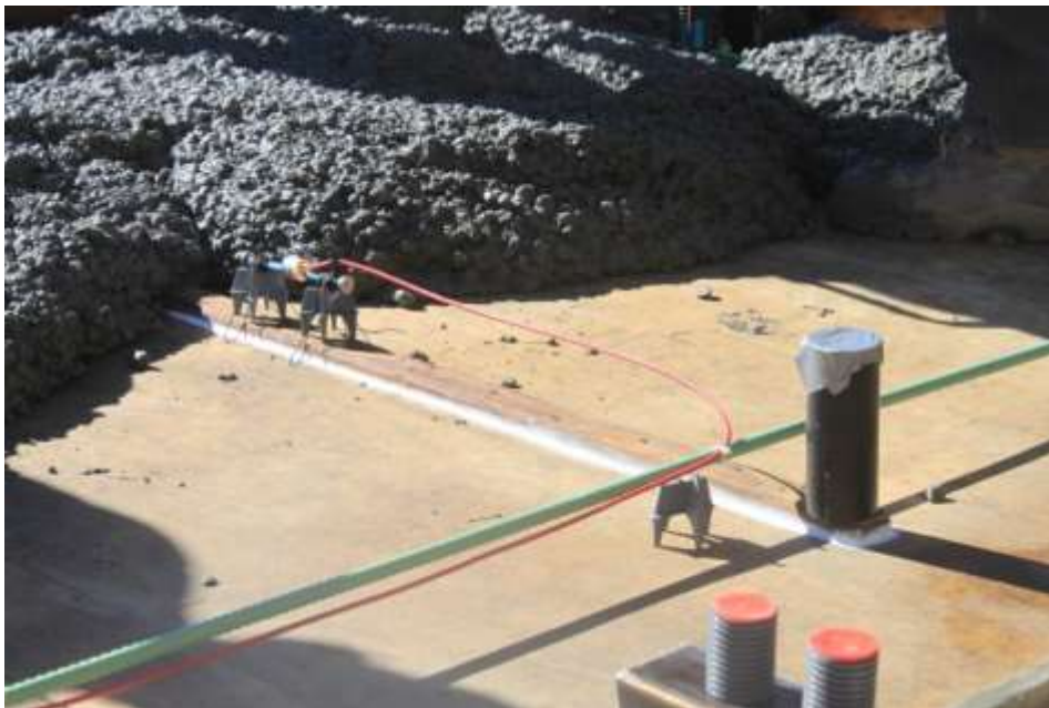
Figure 4: Strain gauge sensor placed in the precast SFRRRC slabs (Abaza, 2016).
