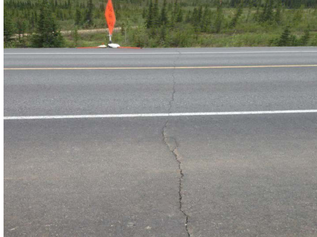
Figure 4.20 Natural transverse crack observed
