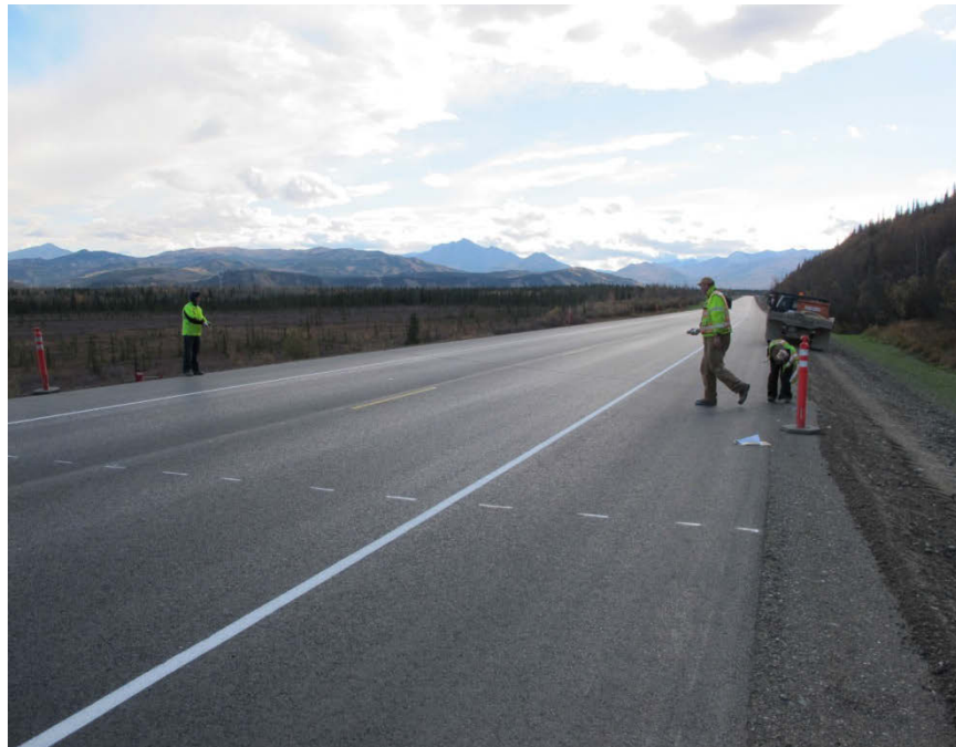
Figure 3.4 Surveyors laying out precuts with rabbit-tracks
