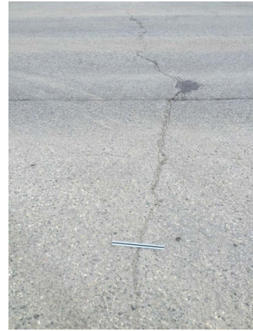
(c) Transverse crack
