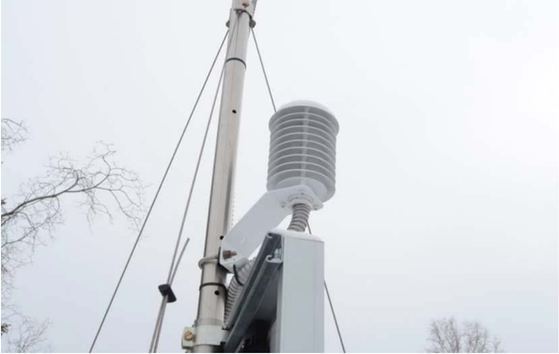
Figure 5.7 Air Temp/Relative Humidity sensor
