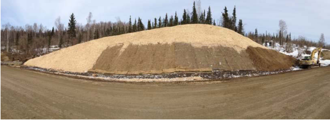
Figure 4.26 Appearance of Experimental Feature soon after completion
