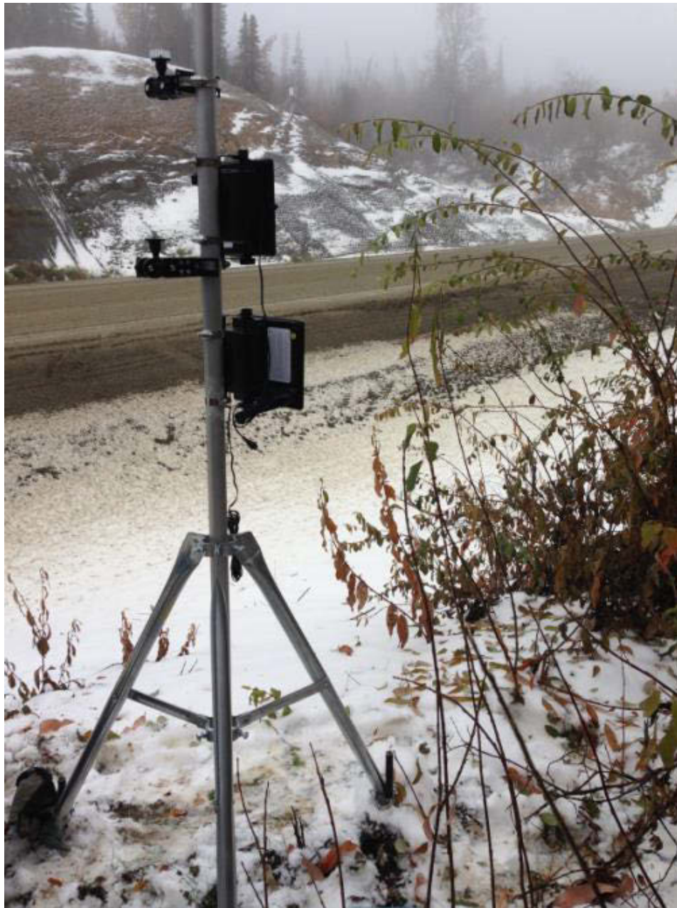
Figure 5.11 Two cameras installed for slope monitoring
