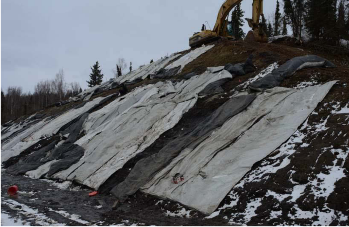
Figure 4.10 Cut slope protected from erosion during drilling
