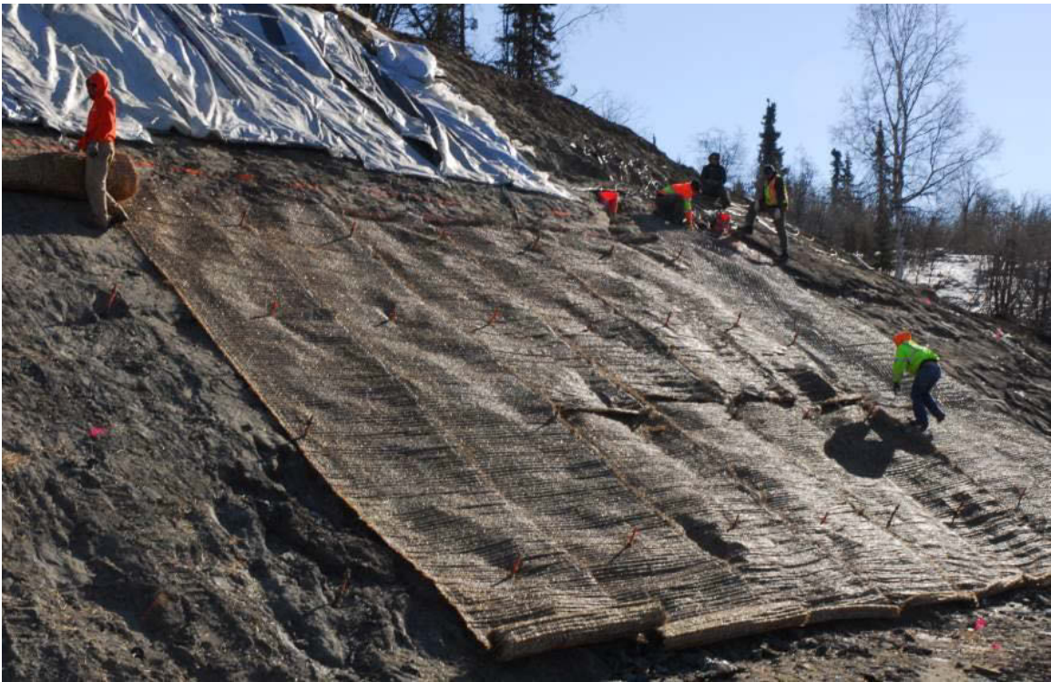
Figure 4.16 Placement of coconut erosion control matting
