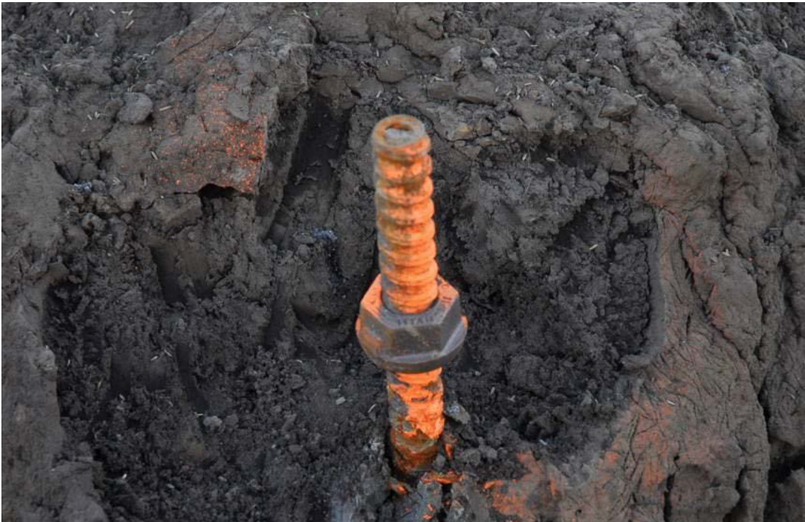
Figure 4.12 Installation of hollow rebar anchor
