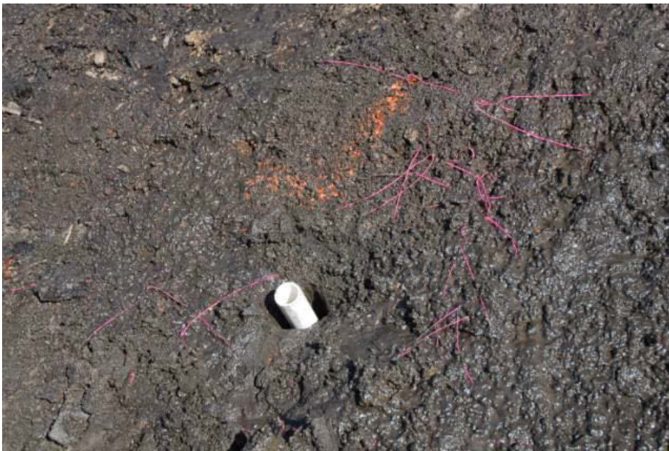
Figure 4.6 Instrumentation hole with sensor housing installed
