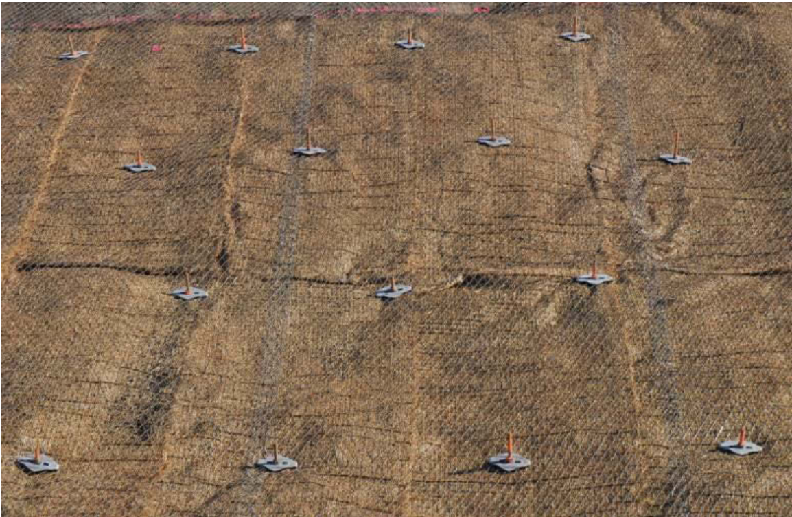
Figure 4.22 Section C appearance after construction
