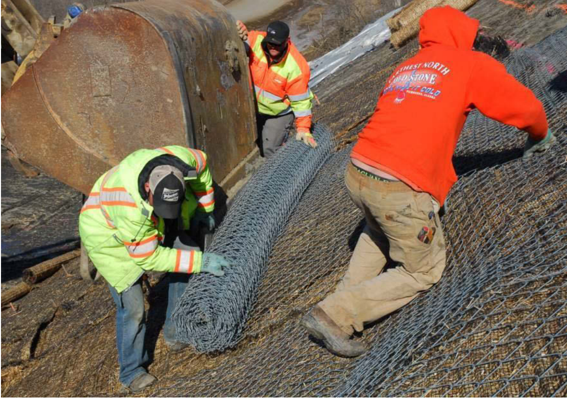
Figure 4.19 Placement of Tecco-mesh
