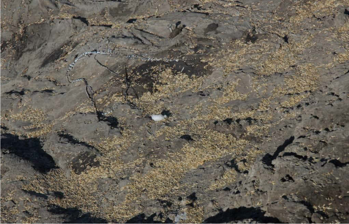
Figure 4.14 Seeded cut slope
