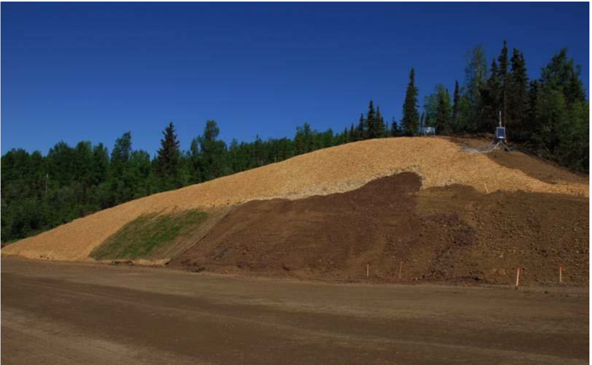
Figure 6.8 Cut slope after construction on Section C
