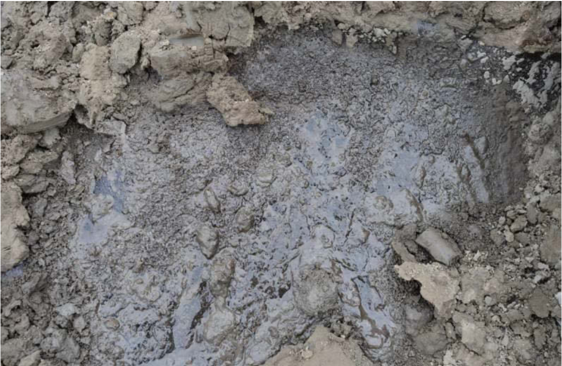
Figure 4.9 Ice exposed in the cut slope
