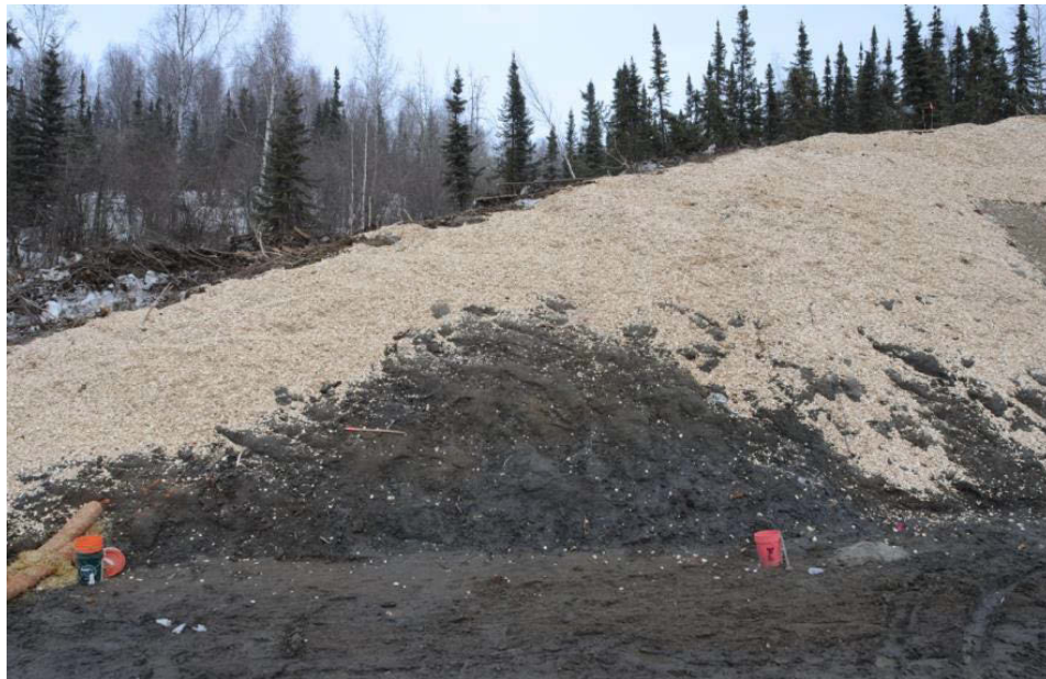
Figure 7.24 Section A after construction on April 26, 2013
