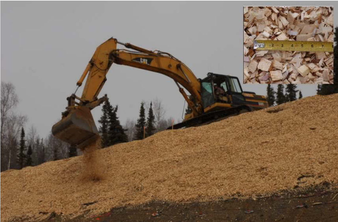
Figure 4.25 Spreading wood chips along top portion of cut slope
