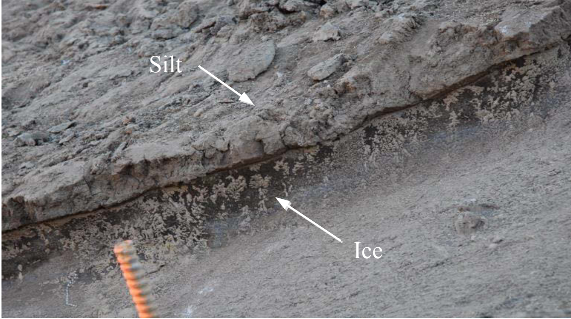
Figure 4.8 Ice in the cut slope
