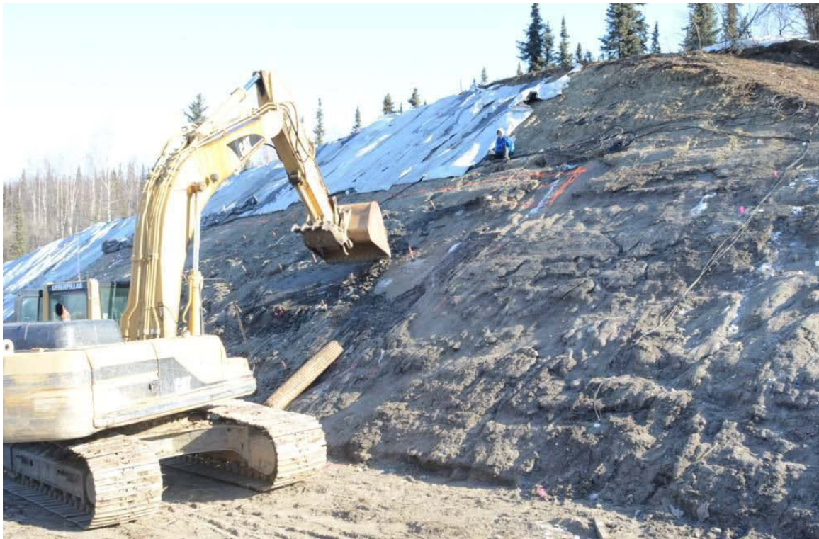
Figure 4.13 Re-smoothing the cut slope surface
