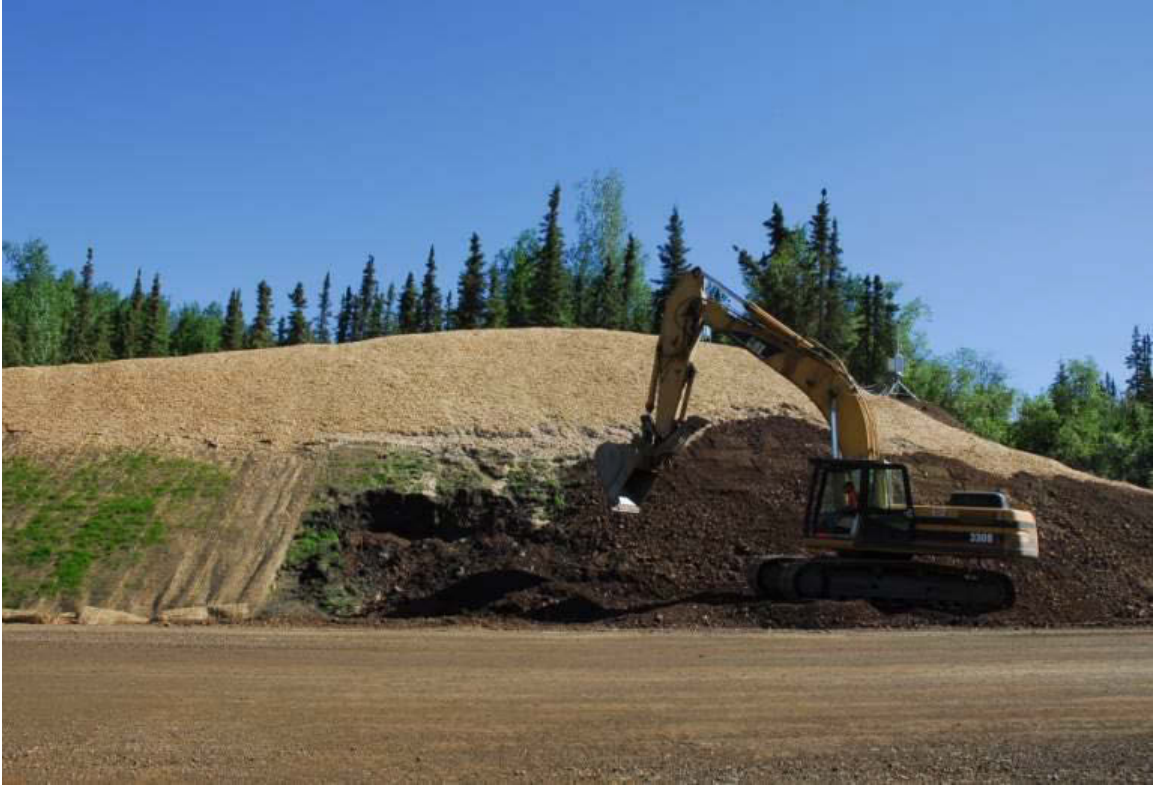
Figure 6.7 Covering Section C with crushed rock
