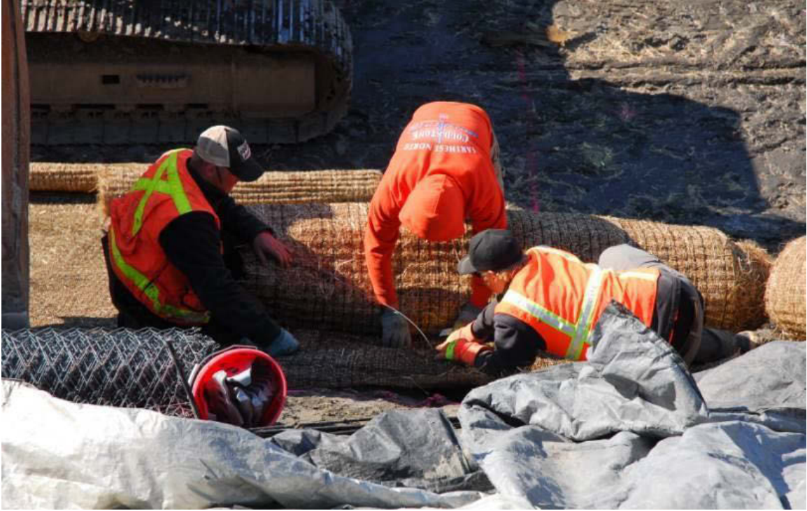
Figure 4.15 Placement of the coconut erosion control matting
