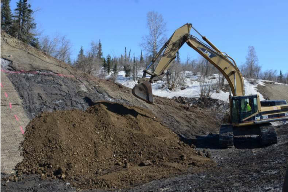
Figure 4.24 Construction of Section D
