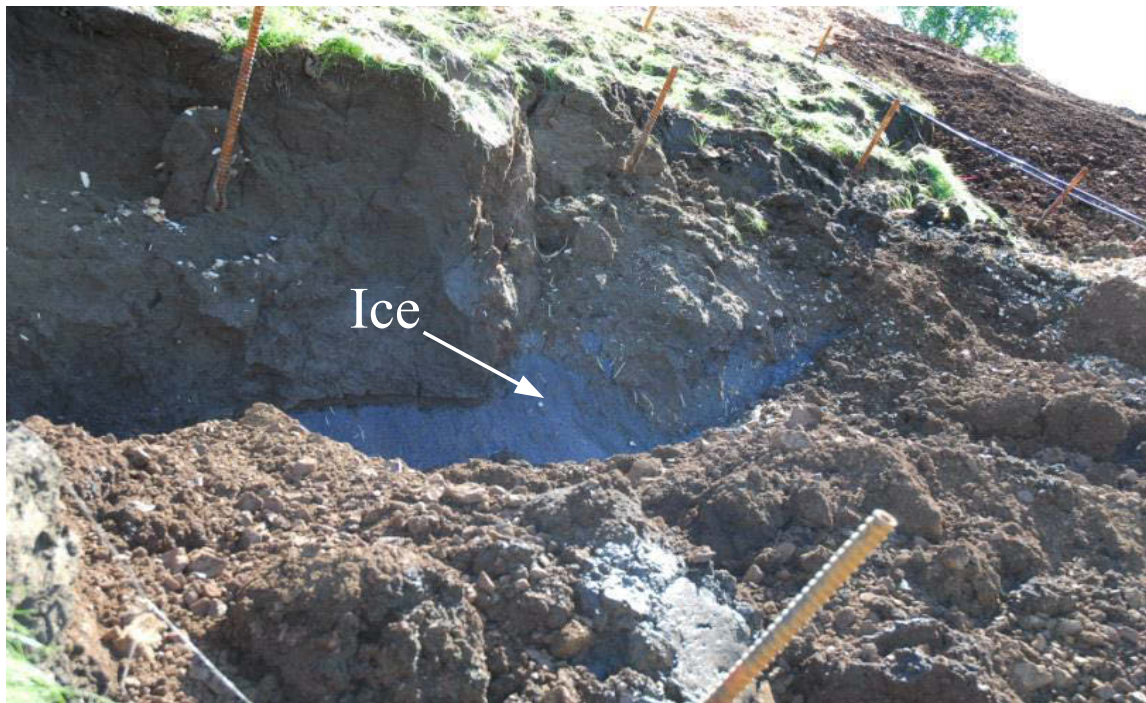
Figure 6.6 Massive ice in Section C
