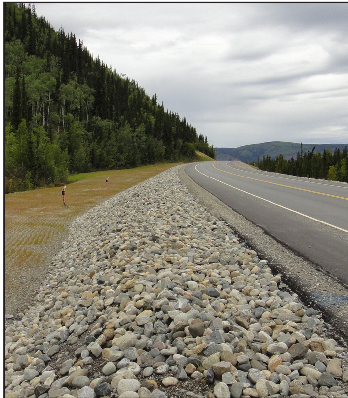
ACE experimental feature on the Alaska Highway at MP 1354–1364. On the left two data loggers gather temperature data year round, which is transmitted to a vendor via satellite.
