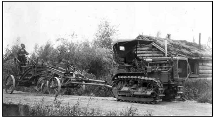
Adams grader and Caterpillar tractor working outside Fairbanks, 1928.
