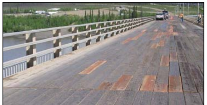
Timber deck repair; a maintenance activity.
