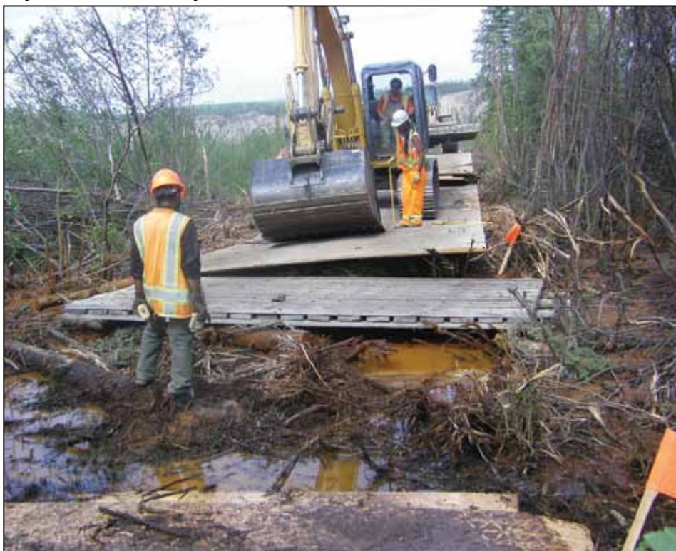
AKDOT&PF maintenance and operations crews install DURA-BASE composite mats for use as a temporary road after Mission Road in Eagle was covered with ice and debris.
