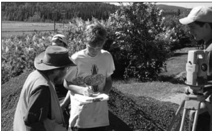
Everett Jorgenson takes careful notes as Thorton DePriest calls out coordinates while using the "total station" for turning corners to ensure the bridge approach is correct.
