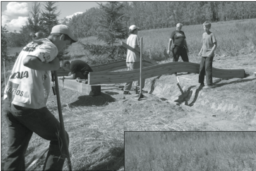
The bridge starts to take shape as the laminated beams are set in place and the layout is checked.
