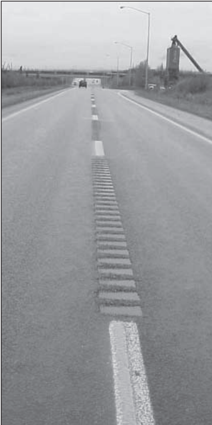
Rumble strips are used on the centerline to help prevent crossover accidents.
