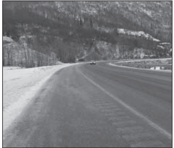
Rumble strips on the Seward highway, a popular road for long haul driving and a good place to stay awake.
