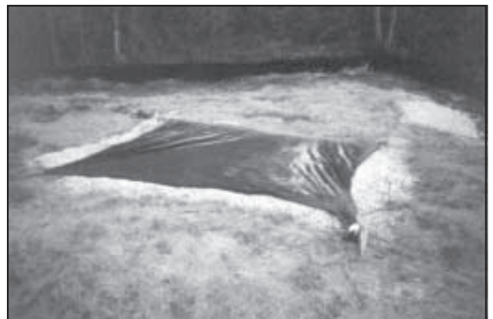
The Georgia DOT has started using geotextile filter bags to trap silt when pumping water from sediment basins and bridge footings.
