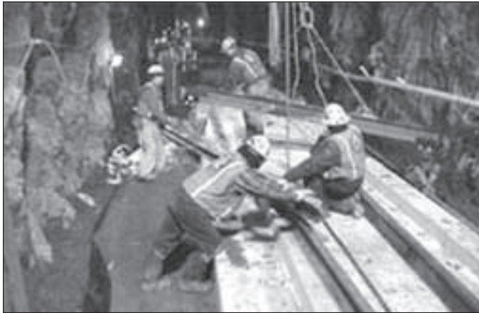
Workers laying rail in the tunnel.
