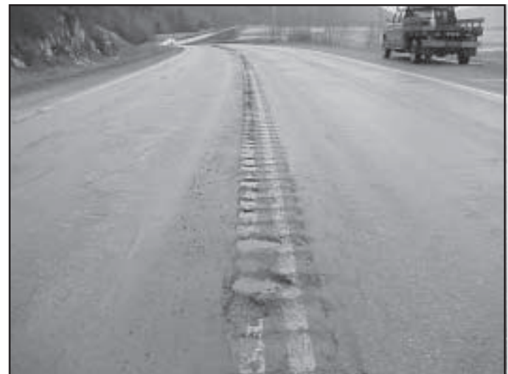
Rumble strips are not problem-free. One problem is accelerated pavement deterioration if rumble strips are installed in marginal or distressed pavements.
