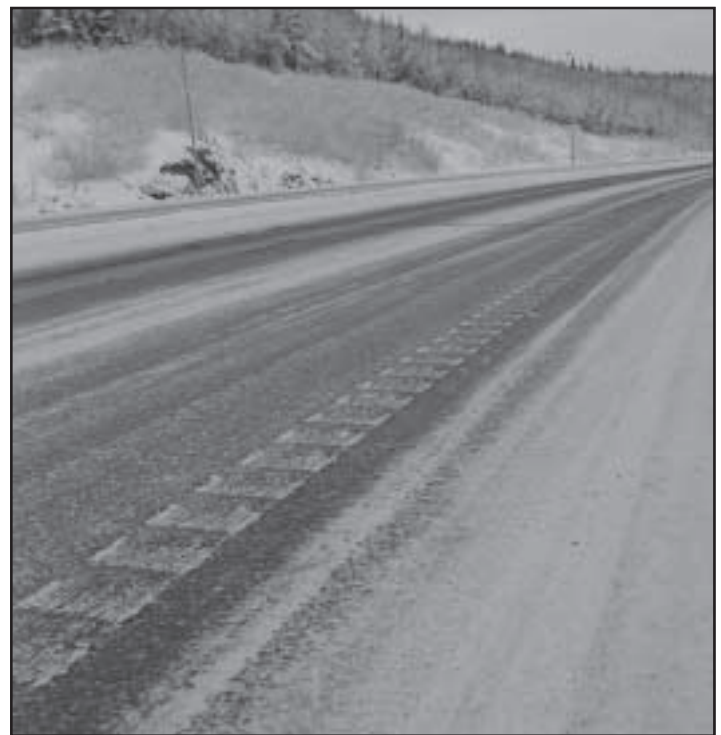
One benefit of rumble strips is enhanced lane delineation during periods when lane striping isn’t visible.
