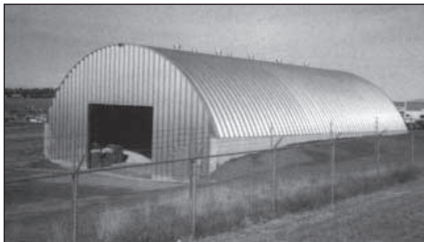
Burleigh County Salt Shed
