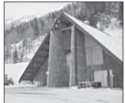
Portal buildings at both ends of the tunnel can withstand avalanche loads up to 1,000 pounds per square foot.
