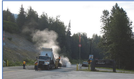
Chip seal crew chip sealing at border with Canada on the Haines Highway. Photo by Ivar Enge, Alaska DOT&PF Southcoast Region.
