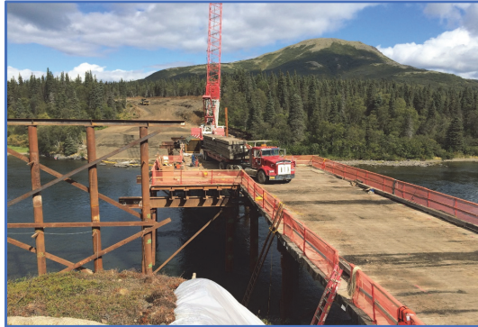
Aleknagik Wood River Bridge Construction, Phase I. Photo by Winnie Cichosz, Alaska DOT&PF
