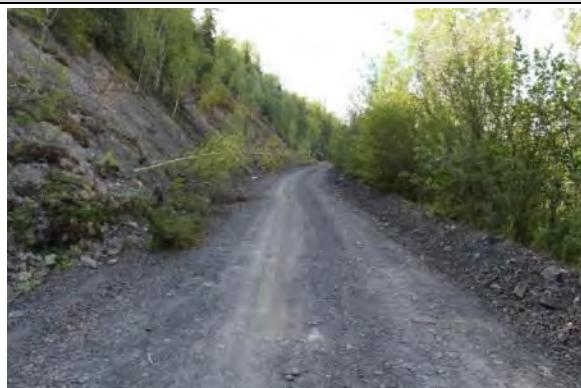
*Figure 30. Gravel roadbed, one travel lane, and embankment reflective of pre-1959 period of significance – south of the Tatralina River. View facing south.*
