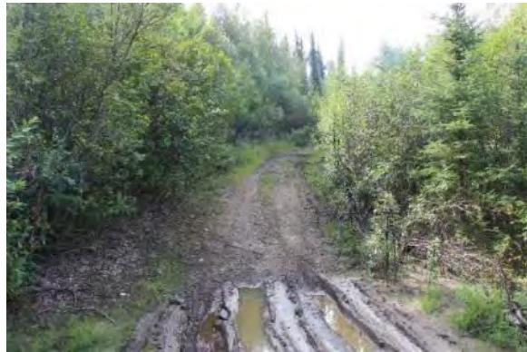
*Figure 28. Example loss of embankment (unmaintained). View facing east.*
