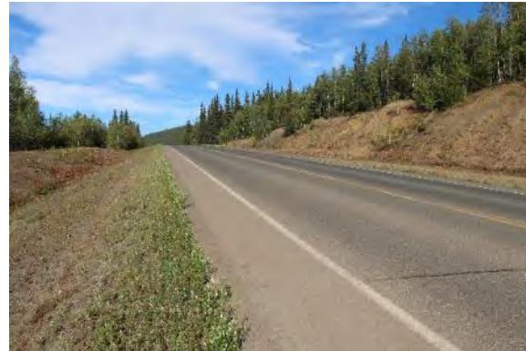
*Figures 10 (view facing southeast) and 11 (view facing northeast). Typical roadbed showing extent of wide embankment.*
