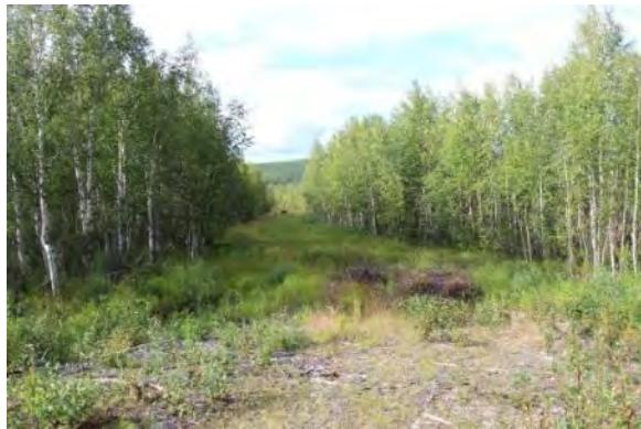
*Figure 25. Example loss of embankment and travel lanes (obliteration of roadbed). View facing north.*
