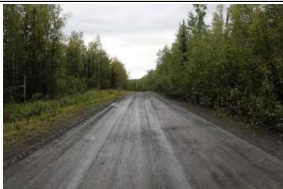
*Figure 29. Gravel roadbed, two travel lanes, and embankment reflective of pre-1959 period of significance – south of the Tatralina River. View facing east.*
