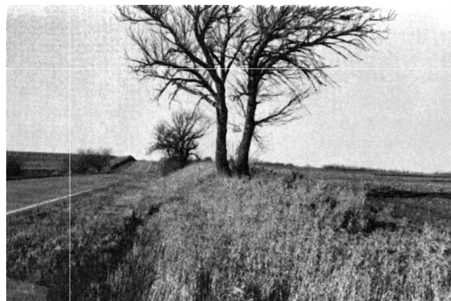
Figure 1160-4 Rural Roadside Hazard Rating of 4
