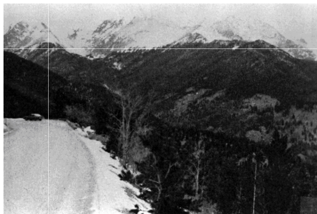
Figure 1160-7 Rural Roadside Hazard Rating of 7
