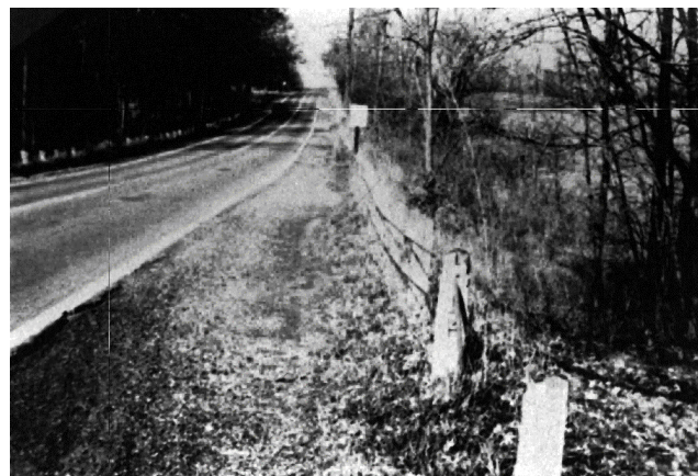
Figure 1160-5 Rural Roadside Hazard Rating of 5
