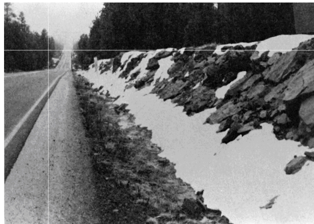
Figure 1160-6 Rural Roadside Hazard Rating of 6
