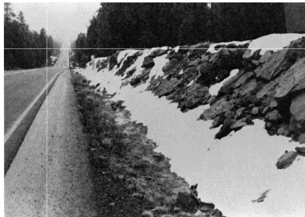
Figure 1160-6 Rural Roadside Hazard Rating of 6
