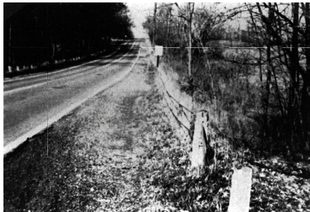
Figure 1160-5 Rural Roadside Hazard Rating of 5
