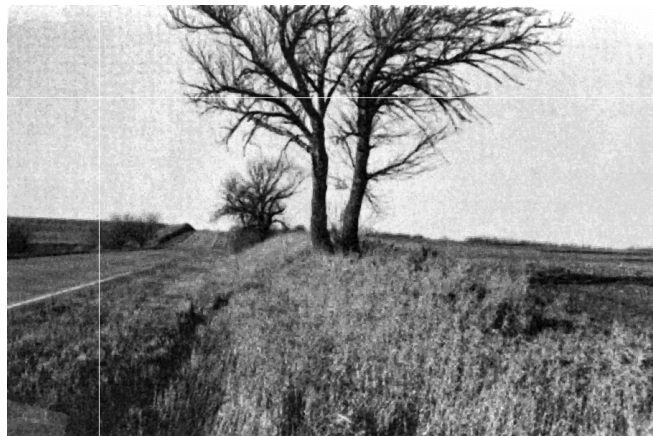
Figure 1160-4 Rural Roadside Hazard Rating of 4
