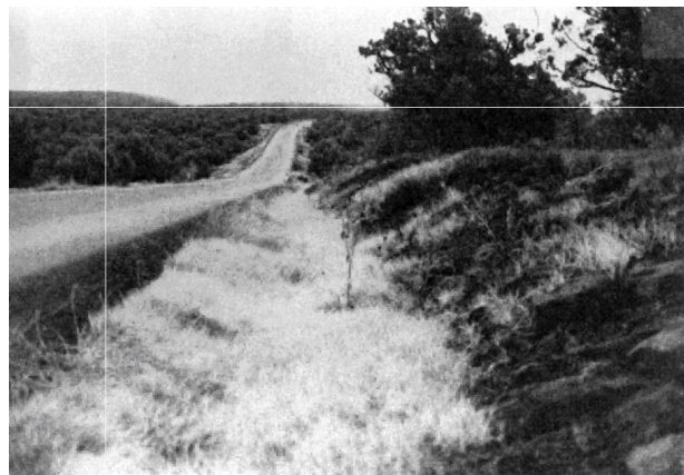
Figure 1160-3 Rural Roadside Hazard Rating of 3
