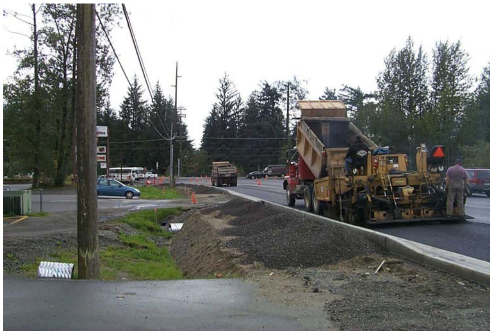
Figure 6-1 Truck Dumping into Paver
