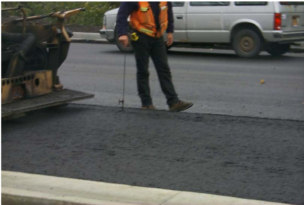
Figure 6-4 Checking Pavement Thickness
