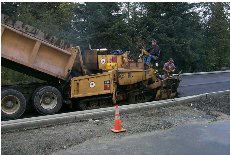
Figure 6-8 Paver in Operation
