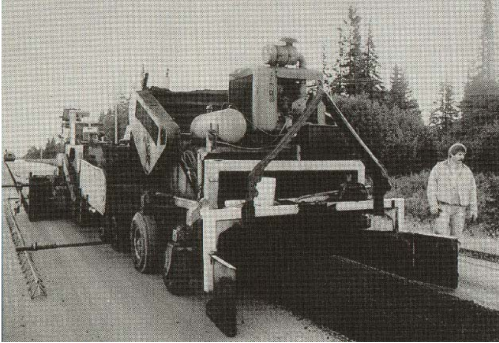
Figure 6-5 Pickup Machine and Paver
