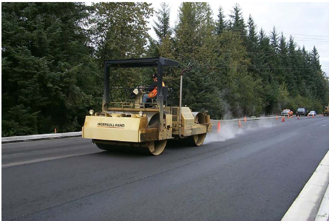
Figure 6-6 Steel Wheel Roller
