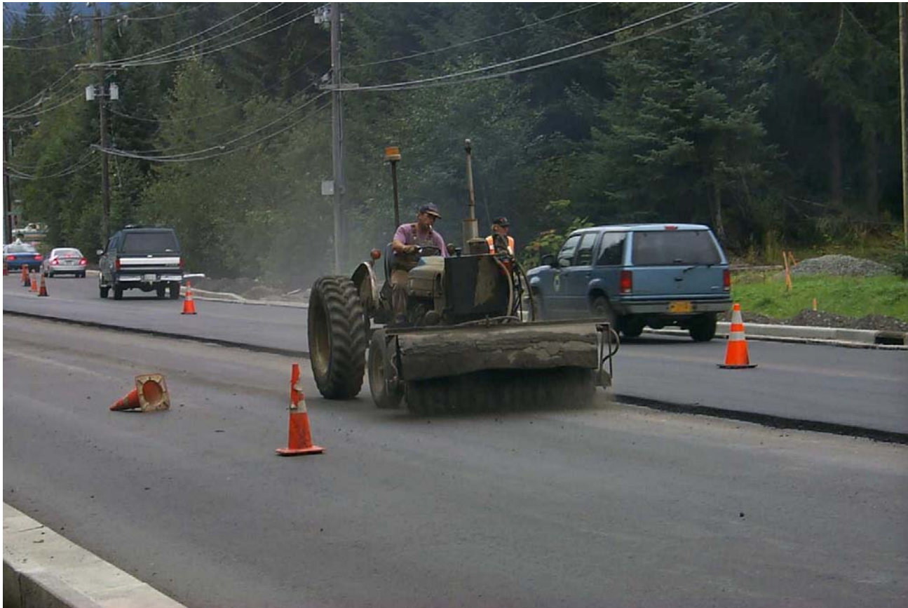
Figure 5-1 Power Brooming Before Tacking
