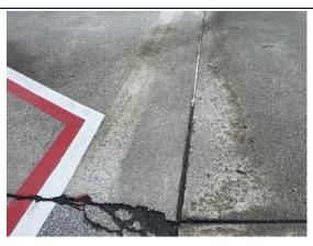
The PCC section consists of a single hardstand constructed in 1997. No major work has occurred since that time. The most common distresses observed are low severity joint and corner spalling, low severity scaling, and medium severity joint seal damage. Field observations indicate that the concrete has several spalls across the hardstand and the joint sealant is failing in areas.
