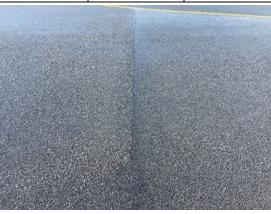
The general aviation parking apron was constructed in 1997 and received a 2-inch overlay in 2015. The most common distresses observed are low severity longitudinal and transverse cracking, low to high severity raveling, and oil spillage. Field personnel noted that the longitudinal paving lane joints are degraded, which is causing longitudinal cracking and raveling to develop.
