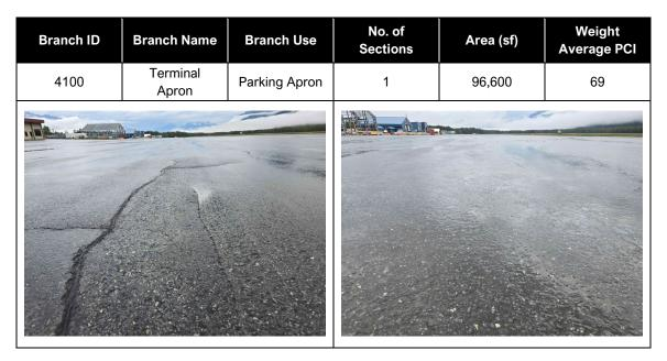
The Terminal Apron was originally constructed in 1981 and was resurfaced in 2006. Commonly observed distresses are low to medium severity longitudinal and transverse cracking, low to medium severity weathering and low severity raveling. There are isolated areas of medium severity raveling.
