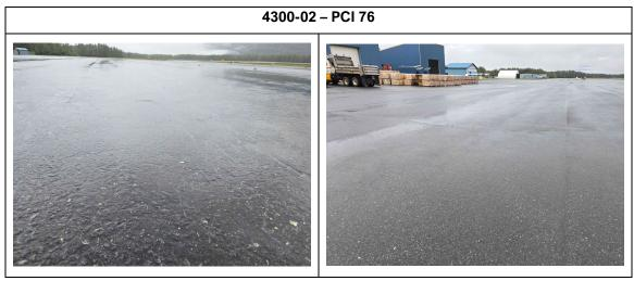
The second section of the West Apron is 4300-02, which was constructed in 1976 and resurfaced in 2006. Observed distresses are low severity longitudinal and transverse cracking, low to medium severity weathering and low severity raveling. There are scattered areas of medium severity raveling from snowplow damage.
