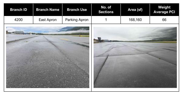
The East Apron was constructed in 1974 and resurfaced in 2006. Observed distresses are low to medium severity longitudinal and transverse cracking, low severity weathering and low severity raveling. There are scattered areas of medium severity weathering and medium severity raveling across the apron.
