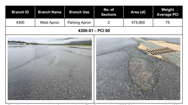
The West Apron consists of two sections. The first section, 4300-01, was constructed in 1981 and resurfaced in 2006. Observed distresses are low to medium severity longitudinal and transverse cracking, low to medium severity weathering and low severity raveling. There are scattered areas of medium severity raveling, with an area of high severity raveling and patching around the drain pictured above.
