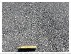
Terminal Apron Section 4100-02 was constructed in 2003 and has not received any major work since. Crack seal operations have not been performed on the section. The most common distresses observed are low severity longitudinal and transverse cracking, oil spillage, low to medium severity raveling, and low to medium severity weathering. Field observations include continued deterioration to the top layer of AC, leading to increased loss of the fine and coarse aggregates across the apron.
