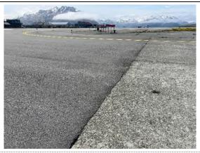
Taxiway B is comprised of two sections, Section 0200-01 and Section 0200-02. APC Section 0200-01 was originally constructed in 1943 using PCC and has undergone multiple AC surface rehabilitations over the years, with the most recent occurring in 2014. Crack seal operations have not been performed on the section. The most common distress observed is low to medium severity weathering. Field observations include initial deterioration to the top layer of AC.
