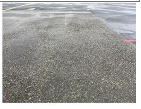
The three PCC sections consist of three separate hardstands. Section 4 was constructed in 1983 and Sections 5 and 6 were constructed in 2012. No major work has been conducted on these PCC sections. The most common distresses observed are medium to high severity joint and corner spalling, low to high severity scaling, and high severity joint seal damage. The concrete is showing its age at nearly 40 years old with numerous high severity distresses.
