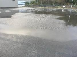
The Northwest Taxi Lane was constructed in 2002 and has not received any major work since. The most common distresses observed are low to medium severity depression, low severity longitudinal and transverse cracking, and low severity raveling. Field observations include the degradation of the paving joints causing longitudinal cracking and raveling. In addition, we observed a number of large areas of depressions, as evidenced by significant areas of standing water.
