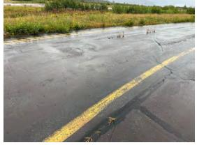
Sections 200-01 and 200-02 of Taxiway B were constructed in 1975 and resurfaced in 1983. Common distresses include low to medium severity longitudinal and transverse cracking, low severity weathering, and low to medium severity raveling. Other distresses observed include depressions, alligator cracking, rutting and swelling of varying severities.
