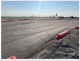
Taxiway A was first constructed in 1993 and was under construction during the 2024 inspection due to a runway realignment project. The project includes removal of the existing asphalt pavement and placing 4" of P-401 HMA on top of 6" of P-209 CABC. Construction was ongoing during the inspection, as paving operations on the taxiway had yet to commence. However, the project will be finished by the end of the 2024 construction season.
