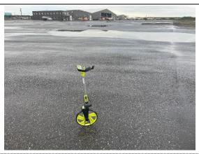
Main Apron Section 4100-06 was constructed in 1971 and has been rehabilitated in 2002 and again in 2015. The most common distresses are low to high severity depressions, low to medium severity longitudinal and transverse cracking, and low severity raveling. Pavement inspectors observed aircraft operators taking measures to avoid several large high-severity depressions on the parking apron. High-severity depressions indicate a significant loss of support.
