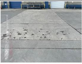
PCC Section 4100-07 of the Main Apron was initially constructed in 2001 and was completely reconstructed in 2019. The most common distresses are low severity joint seal damage and low to medium severity joint spalling. Pavement inspectors note that longitudinal and transverse joints are becoming worn.
