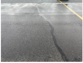
Taxiway E was initially constructed in 1971 and consists of four sections. The most recent major work was rehabilitation in 2022, concurrent with the foamed asphalt stabilized base project performed on Runway 3/21. Crack sealing has been performed annually on the branch. The most common distress is low severity longitudinal and transverse cracking. Field observations include the start of reflective cracking through the recent overlay.
