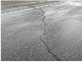
Taxiway E Section 0500-02 was reconstructed in 2015. Crack sealing has been performed annually on the branch. The most common distresses are low severity depressions, low to medium severity longitudinal and transverse cracking, and low severity raveling. Field observations indicate cracks beginning to depress, increasing the severity of the cracking distress. Moreover, localized areas of raveling can be observed adjacent to the paving lane joints.
