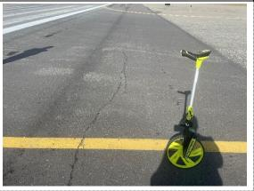
Taxiway G Section 0700-02 underwent major rehabilitation in 2023, concurrent with the foamed asphalt stabilized base project performed on Runway 10/28. Crack sealing has been performed annually on the branch. The most common distress is low severity longitudinal and transverse cracking. Field observations include the initiation of reflective cracking through the recent overlay.
