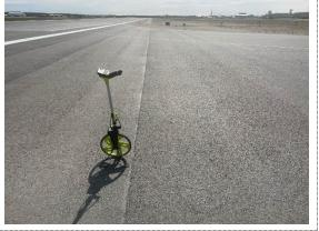
Taxiway F Section 0600-02 underwent major rehabilitation in 2023, concurrent with the foamed asphalt stabilized base project performed on Runway 10/28. Crack sealing has been performed annually on the branch. Pavement inspectors observed no distresses on this section.
