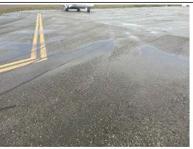
Taxiway J Section 1000-02 has not received any major work since its initial construction. Crack sealing has been performed annually on the branch. The most common distresses are low severity block cracking, low severity depressions, low to medium severity longitudinal and transverse cracking, low severity raveling, and low severity weathering. Pavement inspectors noted that cracks are becoming interconnected and that the area of block cracking appears to be expanding.
