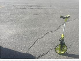
The North Ramp Section 4300-02 was constructed in 1998 and received major rehabilitation in 2015. The most common distresses are low severity depressions, low to medium severity longitudinal and transverse cracking, oil spillage, low to high severity raveling, and low severity weathering. Standing water was observed in depressions on the parking apron. In addition, widespread cracking is beginning to develop and the section would benefit from crack sealing.
