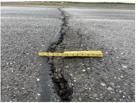
Section 0500-03 of Taxiway E was also reconstructed in 2015. Crack sealing has been performed annually on the branch. The most common distresses are low severity depressions, low to high severity longitudinal and transverse cracking, and low severity raveling. Field observations indicate a high severity transverse crack spanning the entire width of the taxiway, which is depressed and is allowing water infiltration.
