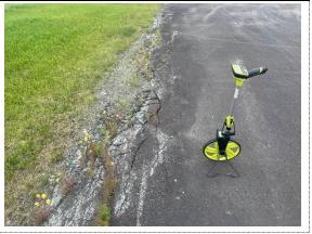
The Compass Rose Apron has not undergone any major work since its initial construction in 1997. Crack sealing has occasionally been performed on the branch. The most common distresses are low to high severity longitudinal and transverse cracking, low to high severity raveling, and low severity weathering. This pavement is degraded and vegetation has grown through most cracks. Furthermore, the pavement edge on the perimeter of the apron is cracked in numerous locations.
