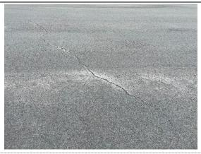
Taxiway G consists of four sections, Sections 0700-01 to 0700-04. Section 0700-01 was completely reconstructed in 2018. Crack sealing has not been performed on section 0700-01. The most common distresses are low to medium severity longitudinal and transverse cracking and low severity weathering. New unfilled cracks have formed and exhibit initial surface deterioration.
