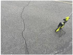
Taxiway N Section 1400-03 was milled and overlaid in 2010. Crack sealing has not been performed on the section. The most common distresses are low to medium longitudinal and transverse cracking and low severity weathering. Pavement inspectors observed an unfilled crack that spans the width of the taxiway.
