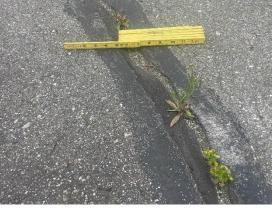
No major work has been performed on Transient Apron 1 since its initial construction in 1978. Crack sealing has occasionally been performed on the branch. The most common distresses are low to medium severity block cracking, low to medium severity longitudinal and transverse cracking, oil spillage, low severity raveling, and low severity weathering. Inspectors noted that while the pavement is cracked, most cracks have been sealed. Vegetation is protruding through the sealant in many instances.
