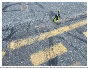
No major work has been performed on Taxiway G Section 0700-04 since its initial construction in 1980. Crack sealing has occasionally been performed on the section. The most common distresses are low to medium severity fatigue cracking, low severity block cracking, medium severity longitudinal and transverse cracking, low severity raveling, and low severity weathering. The pavement surface of this section is highly degraded with a large quantity of load-related distresses throughout.
