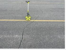
Taxiway B Sections 0200-04 and 0200-05 have not undergone any major work since their initial construction in 2006 and 2017, respectively. Crack seal operations have not been performed on these sections. The most common distresses are low to medium severity longitudinal and transverse cracking, low severity raveling, and low severity weathering. Unsealed longitudinal and transverse cracks have the potential to allow vegetative growth similar to the remainder of Taxiway B.
