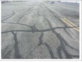
Taxiway Q Section 1700-01a has not undergone any major work since its initial construction in 1997. Crack sealing has occasionally been performed on the section. The most common distresses are low to medium severity block cracking, low severity raveling, and medium severity weathering. The pavement is fully block cracked and although it has been sealed well, the AC surface is highly degraded, with some coarse aggregate particles dislodged.
