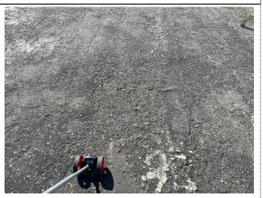
Section 4200-01 of the Retardant Ramp was constructed in 1966 and has not received any major work since. Annual crack seal operations have not been performed on the section. The most common distresses observed are medium severity alligator cracking, high severity block cracking, and medium to high severity raveling. Field observations include a pavement surface that is completely deteriorating away and there is significant FOD potential.
