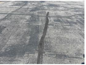
Section 4200-02 of the Retardant Ramp was constructed in 1976 and received a 3-in overlay in 2001. Annual crack seal operations have been performed on the branch. The most common distresses observed are low severity depression, low severity longitudinal and transverse cracking, and low severity weathering. Field observations include wearing of the coal tar treatment leading to the initial loss of the fine aggregate matrix.
