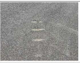
The Main Apron Section 4100-03 was constructed in 2017 and has not received any major work since. Crack seal operations have not yet been performed on the branch. The most common distresses observed are oil spillage, medium to high severity raveling, and low severity weathering. Field observations include the initial wearing of the pavement surface, large areas of oil spillage beginning to soften the asphalt surface, and gouges in the asphalt due to propeller strikes, snow plow operations, etc.
