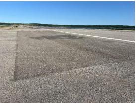
Taxiway D Section 0400-01 was initially constructed in 1975 then received a surface reconstruction along with the runway in 2011. The most common distresses observed are low to medium severity depressions, low to medium severity longitudinal and transverse cracking, low severity patching, and low to medium severity weathering. Field observations include the development of depressions across the taxiway as well as a patched area that is beginning to depress and hold water again.
