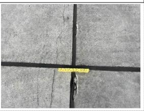
The Main Apron PCC hardstands, Sections 4100-05 and 4100-06, were constructed in 2022 and have not received any major work since. The most common distresses observed are low severity joint seal damage, low to medium severity joint spall, and low severity corner spall. Field observations include minor damage to the joint seal and a few spalls on both hardstands.
