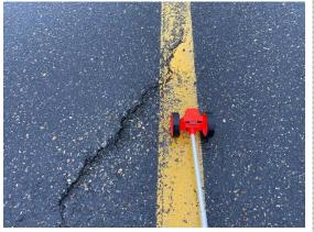
Taxiway F section 0600-03 was initially constructed in 2012 and has not received any major work since. Section 0600-03 connects runway 08/26 with taxiway D. Crack seal operations have not been performed on this section. The most common distresses observed are low to medium severity raveling, and low severity weathering. Field observations include the pavements surface beginning to weather and a few cracks starting to develop.
