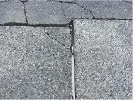
The PCC section 4100-HS consists of two hardstands that were initially constructed in 2001 and there has not been any major work since. The most common distresses observed are low to medium severity joint and corner spalling, low severity scaling, and high severity joint seal damage. Field observations show that the concrete has several spalls across both hardstands and the joint sealant needs replaced.
