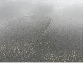
Taxiway C section 0300-02 was initially constructed in 1990 and received surface reconstruction in 2015. Crack seal operations have not been performed on this section. The most common distresses observed are low to medium severity raveling and low severity weathering. Field observations include the pavements surface beginning to weather and a few mechanical gouges from snowplow activities.
