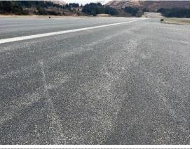
Taxiway E section 0500-01A has the same history as sections 01 and 02 but underwent an additional surface reconstruction concurrently with runway 08/26 in 2012. Crack seal operations have not been performed on this section. The most common distresses observed are low to medium severity raveling, and low to medium severity weathering. Field observations include the pavements surface beginning to weather and localized areas of raveling.
