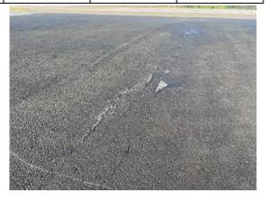
Taxiway C was constructed in 1988. In 2018, the taxiway received a 2-inch overlay. The most common distresses observed are low to medium to high severity raveling, low severity weathering, and bleeding. The weathering and raveling are significant for a 4-year old pavement (at the time of inspection). Also noted were a considerable area of bleeding, which is caused by problems with the asphalt concrete mix properties, such as excessive asphalt binder and/or low air voids.
