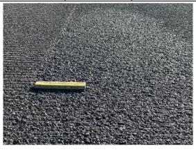
Taxiway B was constructed in 1988 and was reconstructed in 2008. The most common distresses observed are low severity longitudinal and transverse cracking, low to medium severity raveling, and low to medium severity weathering. Our field personnel observed an increased loss of fine aggregate (weathering), which is exposing the coarse aggregate and in some areas the removal of the coarse aggregate altogether (raveling).
