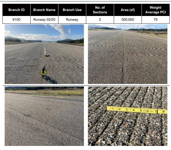
Runway 02/20 was constructed in 1988 and reconstructed in 2008. The most common distresses observed are low severity longitudinal and transverse cracking, low to medium severity raveling, and low to medium severity weathering. We observed the loss of the fine aggregate along the longitudinal construction joints which is exposing the coarse aggregate (weathering) and in some areas the removal of the coarse aggregate altogether (raveling).
