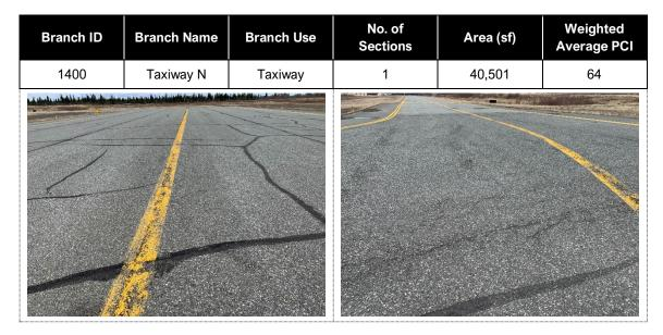
Taxiway N was initially constructed in 1950 and was reconstructed in 2008. Occasional crack seal operations have been performed on the branch. The most common distresses observed are low severity block cracking, low severity longitudinal and transverse cracking, low to medium severity raveling, and low severity weathering. Field observations include localized spots of medium to high severity cracking and medium severity raveling, all near the military taxiway.
