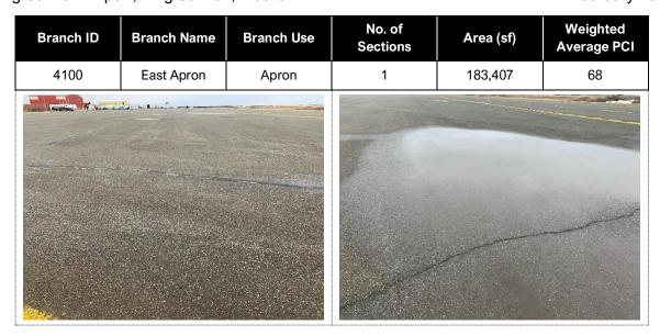
The East Apron was constructed in 1972 and was reconstructed in 2009. The most common distresses observed are low to medium severity depressions, low to medium severity longitudinal and transverse cracking, low severity raveling, and low severity weathering. Field observations include standing water within depressions and the presence of some old crack sealant, although numerous cracks remain unsealed.
