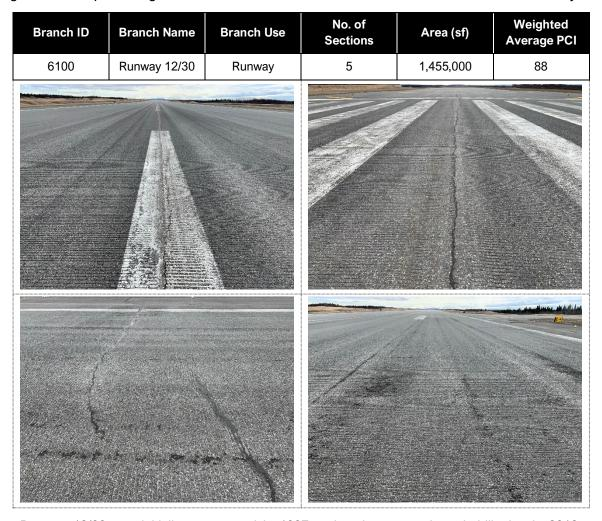
Runway 12/30 was initially constructed in 1997 and underwent major rehabilitation in 2018. Occasional crack seal operations have been performed on the runway. The most common distresses observed are low severity longitudinal and transverse cracking, low severity raveling, and low severity weathering. Field observations include sealed cracks, weathering, and localized areas of raveling. Additionally, low severity depressions are developing in the overrun section near the West Apron.
