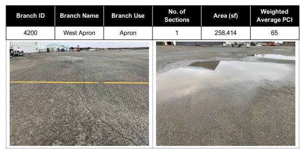
The West Apron was initially constructed in 1991 and was reconstructed in 2009. The most common distresses observed are low to medium severity depressions, low to medium severity longitudinal and transverse cracking, low severity raveling, and low severity weathering. Field observations include standing water within depressions and the presence of some old crack sealant, although most cracks remain unsealed at medium severity level.
