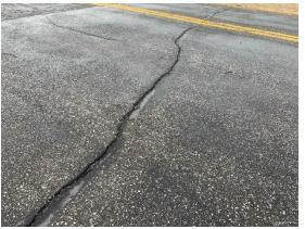
Section 4300-02 (29,159 sq ft) was initially constructed in 1986 and was reconstructed in 2009. Occasional crack seal operations have been performed on the branch. The most common distresses observed are low to medium severity longitudinal and transverse cracking, low severity raveling, and low severity weathering. Field observations include numerous sealed longitudinal and transverse cracks in which some of the sealant is beginning to fail.
