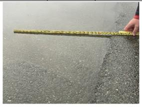
The holding apron was constructed in 1993. The most recent major work conducted on this branch was a 2.5-inch overlay in 2013. The most common distresses observed are low severity longitudinal and transverse cracking, low severity raveling, and low severity weathering. Field personnel observed degradation of the longitudinal construction joints which is causing longitudinal cracking and raveling to develop. Furthermore, dimples were observed across the apron leading to areas of standing water.
