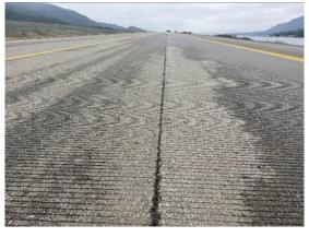
Taxiway B was constructed in 2003 and received a 2.5-inch AC overlay in 2013. The most common distresses observed are low to medium severity longitudinal and transverse cracking, low to medium severity raveling, and low severity weathering. Field personnel observed degradation of the longitudinal construction joints which is causing longitudinal cracking and raveling to develop.
