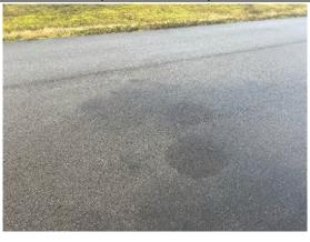
The general aviation apron was constructed in 1970 and was most recently received a 3.0-inch overlay in 2013. The most common distresses observed are low severity longitudinal and transverse cracking, low severity raveling, and oil spillage. Field personnel observed degradation of the longitudinal construction joints, which is causing longitudinal cracking and raveling. Areas of oil spillage were also observed.
