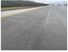
Taxiway A was constructed in 1993. The most recent major work on the taxiway was a 2.5-inch AC overlay in 2013. The most common distresses observed are low severity longitudinal and transverse cracking, low severity raveling, and low severity weathering. Field personnel observed degradation of the longitudinal construction joints which is causing longitudinal cracking and raveling to develop.
